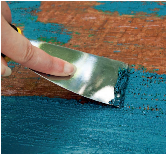
Graffiti cleaning with paint remover
