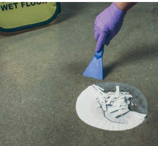
Graffiti cleaning with paint remover
