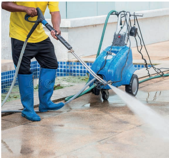
Stain cleaning with high-pressure jet
