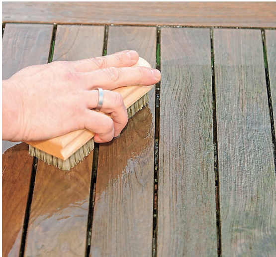
Removing Mould and algae
