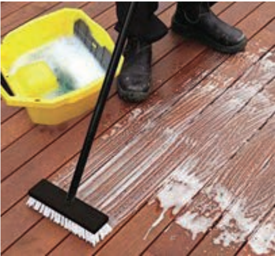
Timber decking cleaning with bristle brush
