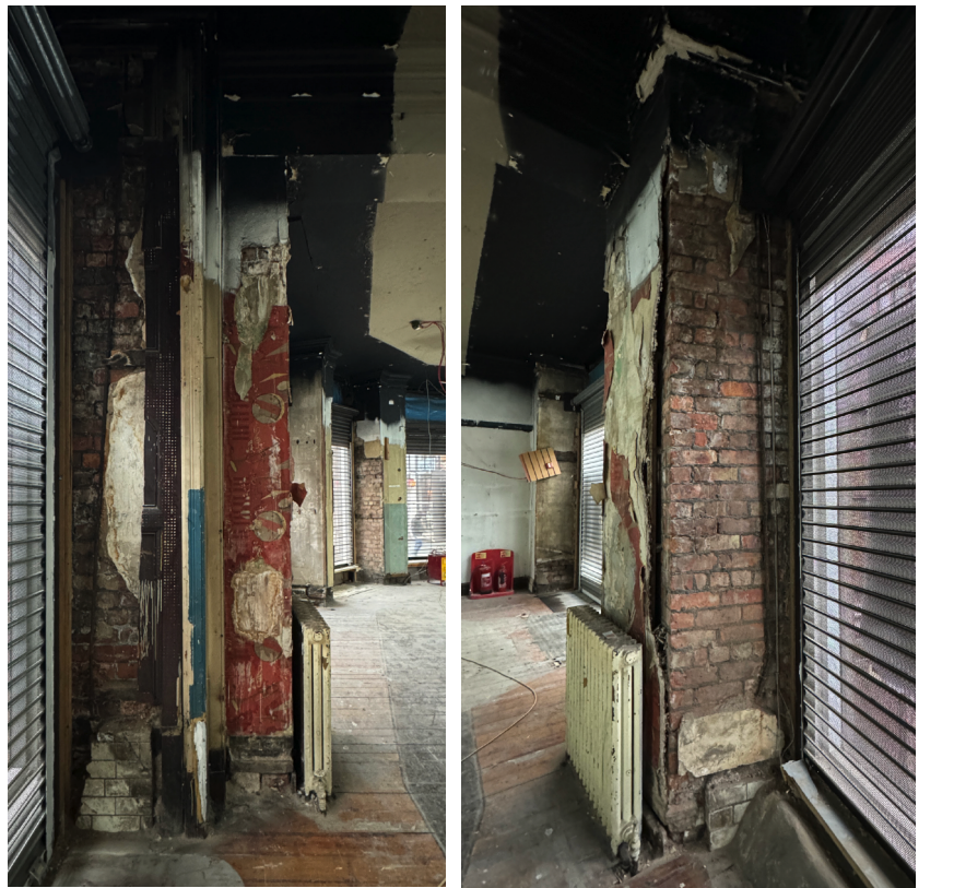
PHOTOGRAPHS SHOWING EXISTING WALL TREATMENT
