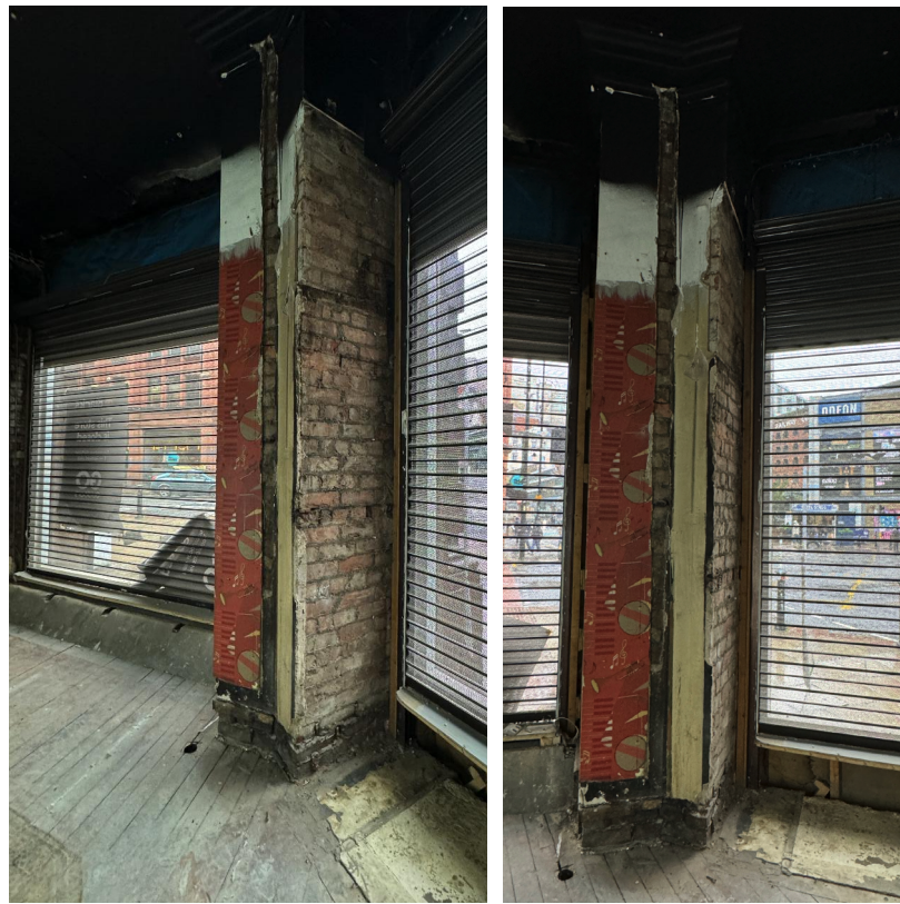
PHOTOGRAPHS SHOWING EXISTING WALL TREATMENT
