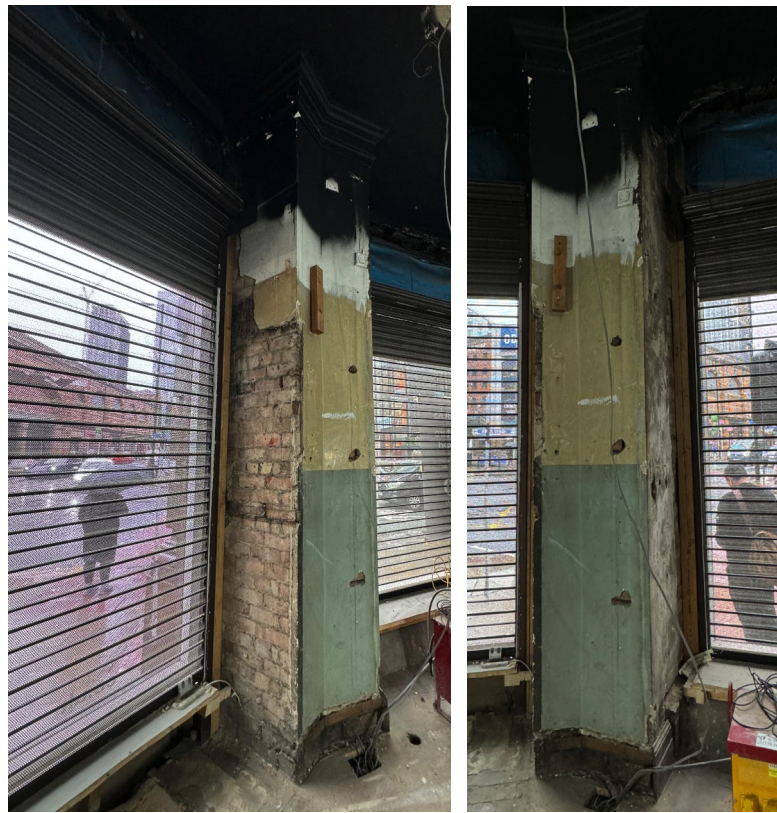
PHOTOGRAPHS SHOWING EXISTING WALL TREATMENT
