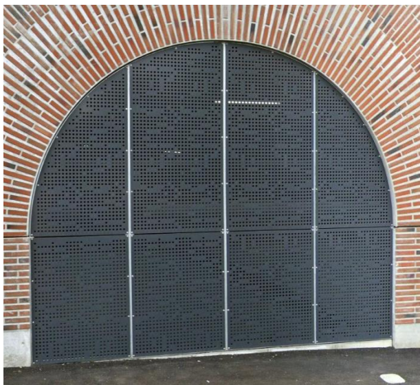
C Vent type C – polyester power coated perforated metal decorative panel
