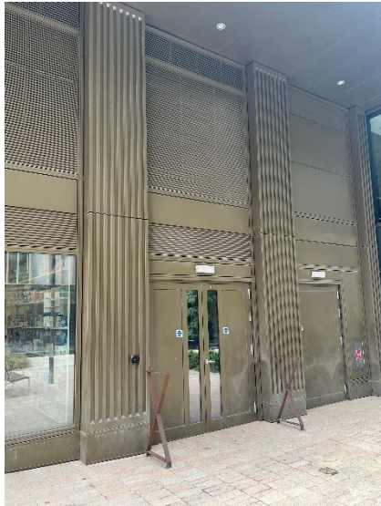
A2 Vent type A2 – polyester powder coated louvre blades, narrow blade profile
