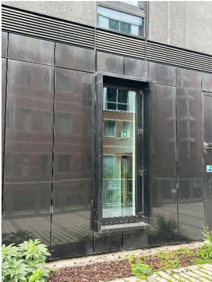
A1 Vent type A1 – polyester powder coated louvre blades, wide blade profile
