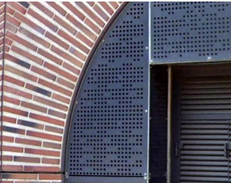
Photograph of perforated metal panels at the MSCP, Circle Square
