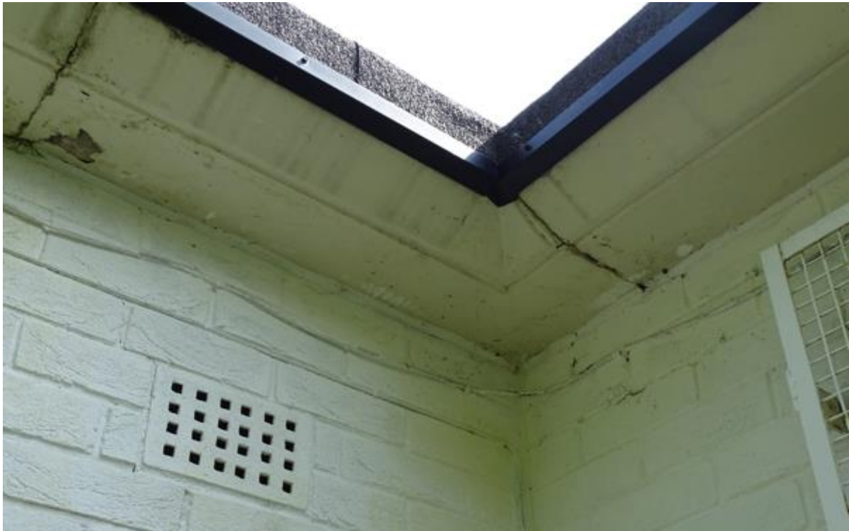
Image 5 – Close view of below flat roof coverings
