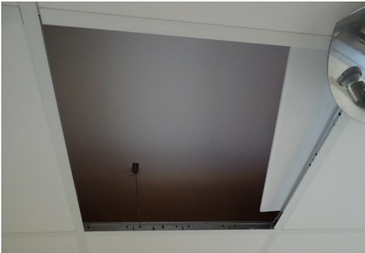
Image 6 – Internal view from below the flat roof coverings
