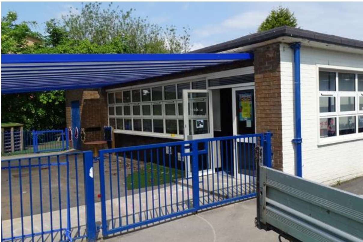
Image 4 – South facing elevation of the structure
