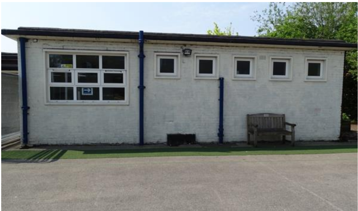
Image 2 – North facing elevation of the structure
