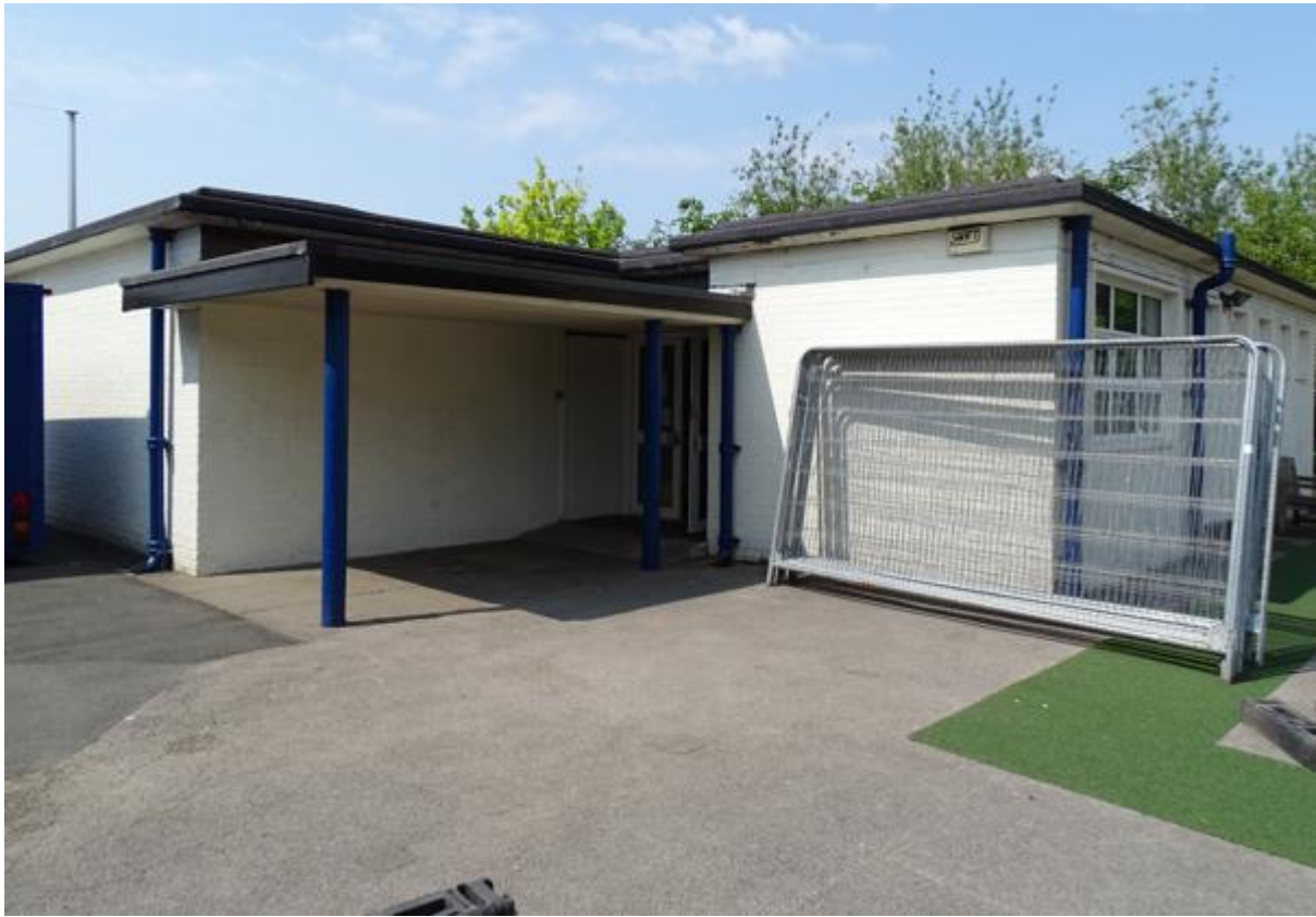
Image 1 – North & East facing elevations of the structure
