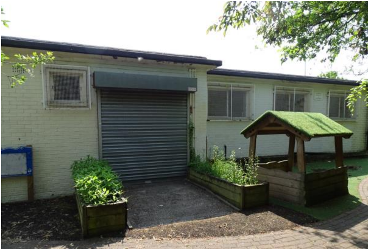
Image 3 – West facing elevation of the structure
