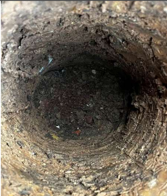
Photograph 1: View of soil in capping layer excavation in front garden of Plot 3.
