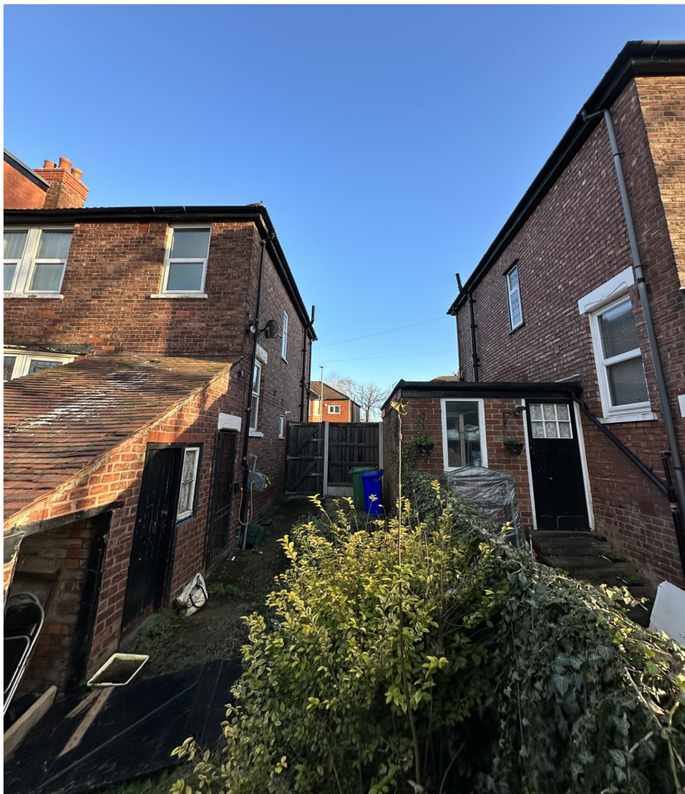
Figure 4. Shared boundary with No.6 Wellington Road.
