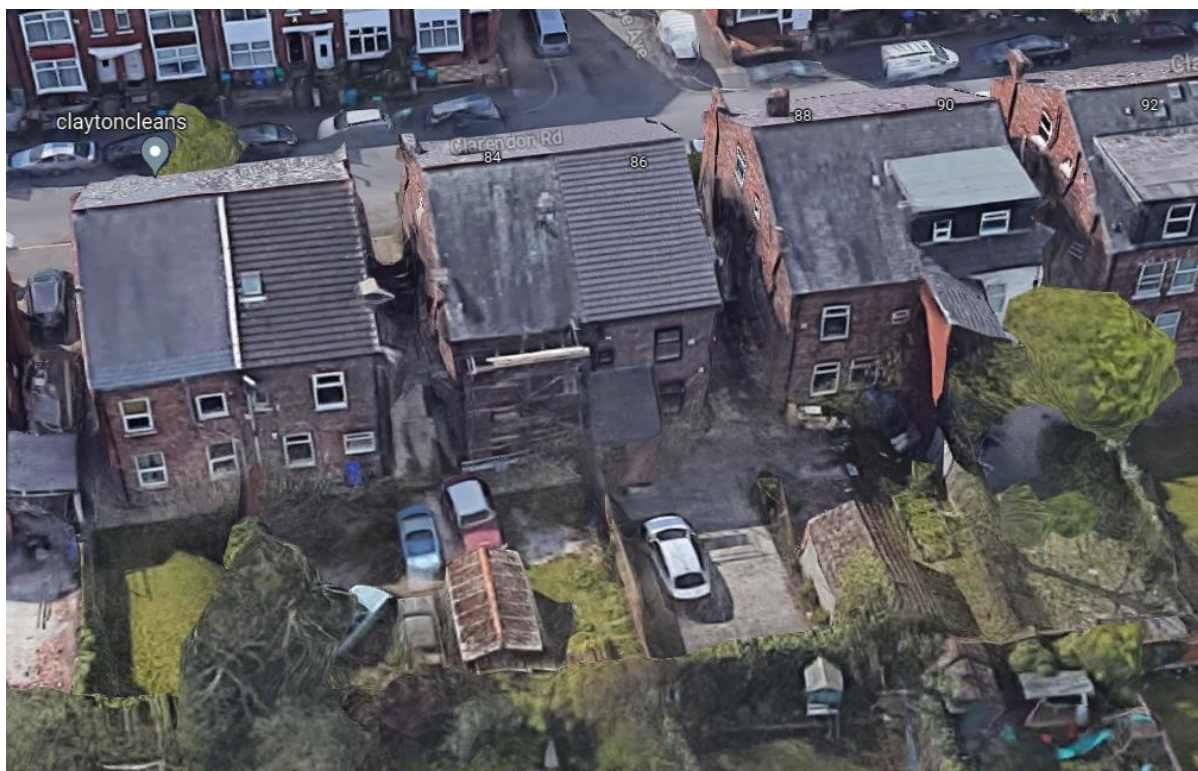
Image 3: Overhead view of the rear of the site currently laid to hardstanding and used for car parking
