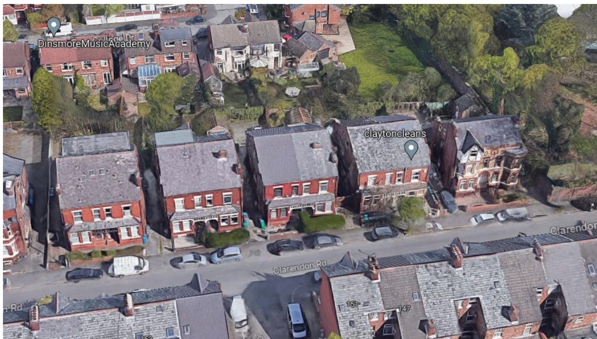
Image 2: Overhead view of the site showing its position within the street scene at the junction of Clarendon Road and Cambridge Avenue
