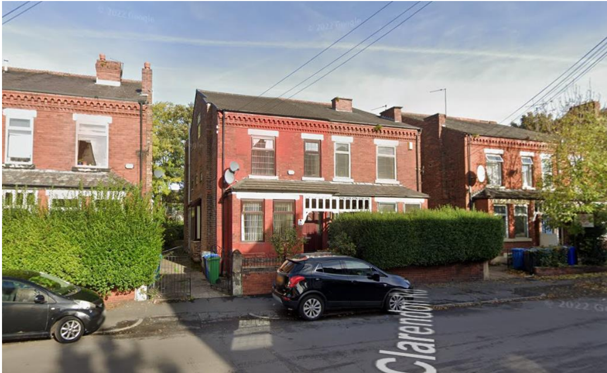
Image 1: The site as viewed from street level with the adjoining semi detached property of No.88 Clarendon Road to the west
