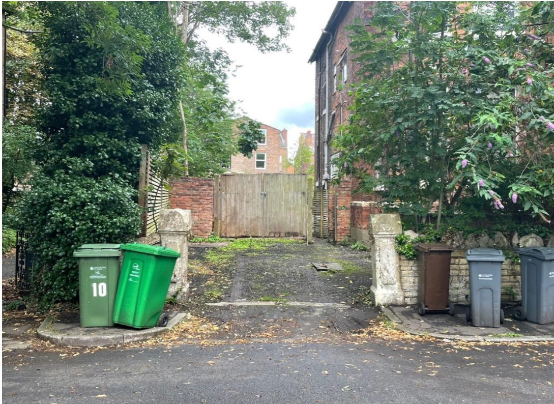
Image 2 – Photograph of vehicular entrance to site from Deerpark Road. Note the untidy refuse arrangement (due to lack of dedicated storage), original gate posts in a state of disrepair, hardstanding to the side of the property and closed boarded gate/fence preventing views of the rear garden beyond.
