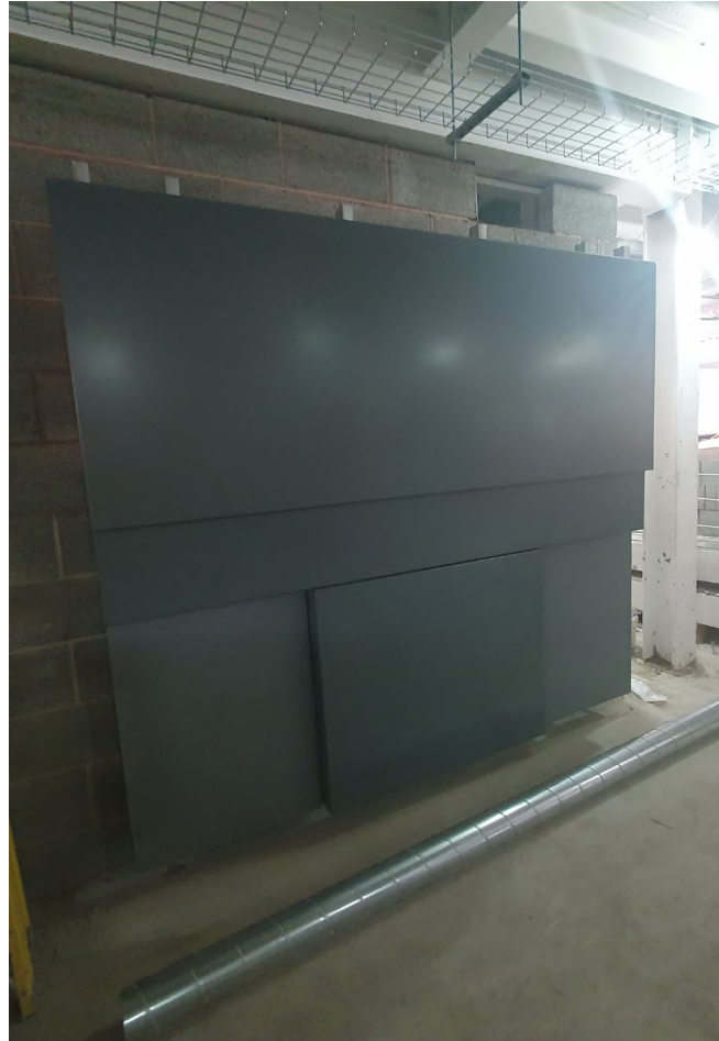
Sample panel images (capping to top edge yet to be added)
