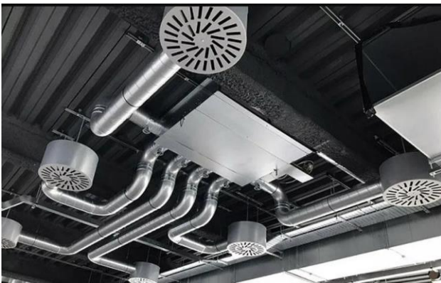
Figure 32 – Typical VRV Fan Coil to Amenity Spaces
