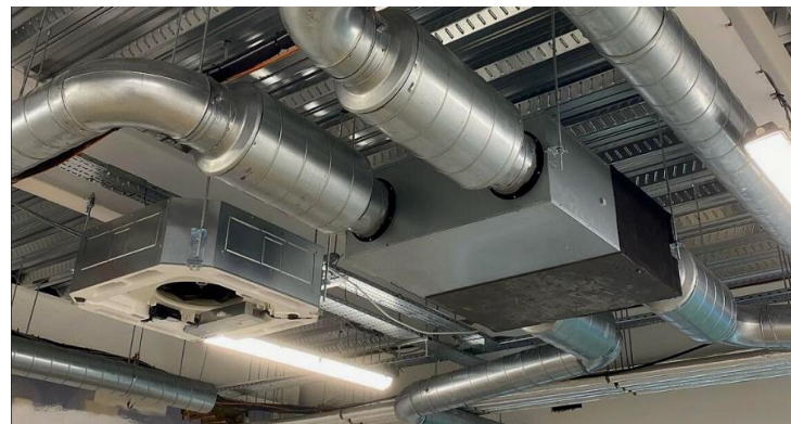
Figure 33 – Typical MVHR Units to Amenity Spaces
