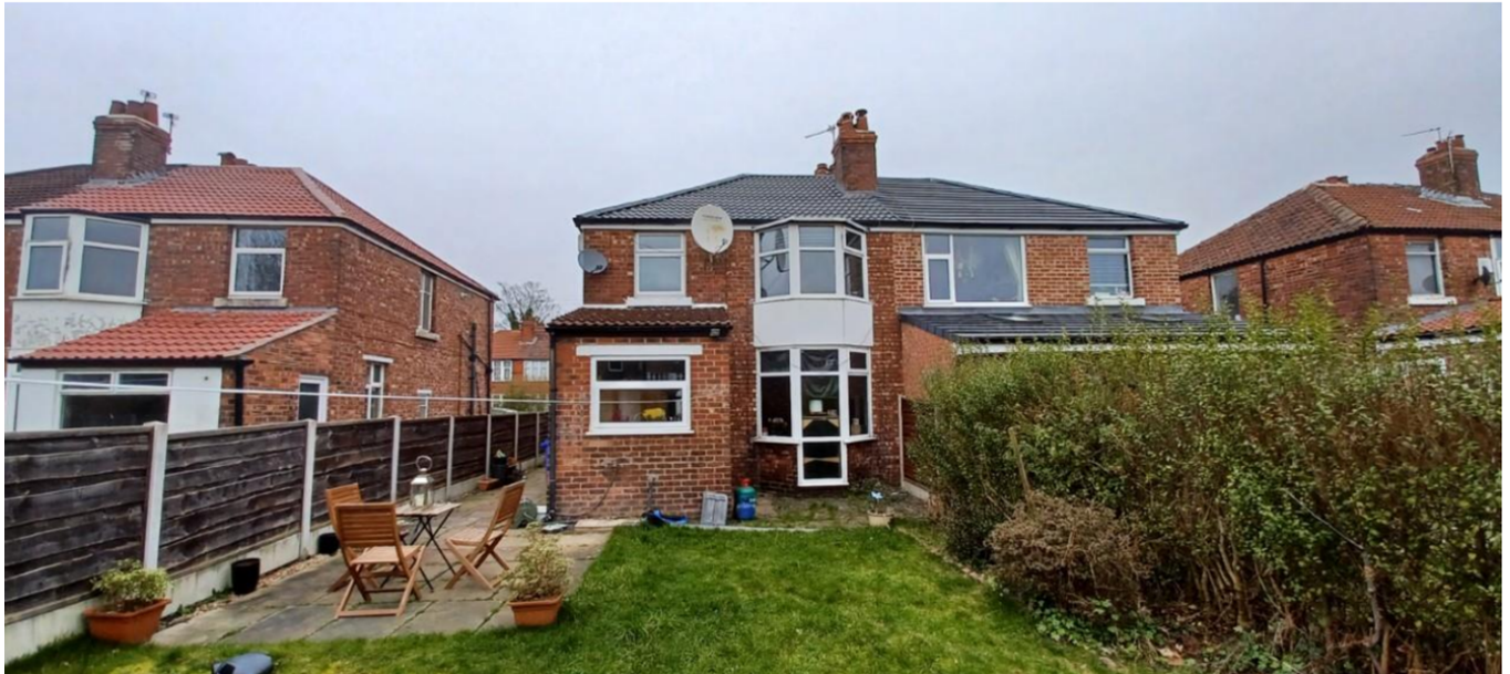
Figure 2. Rear view of property.
