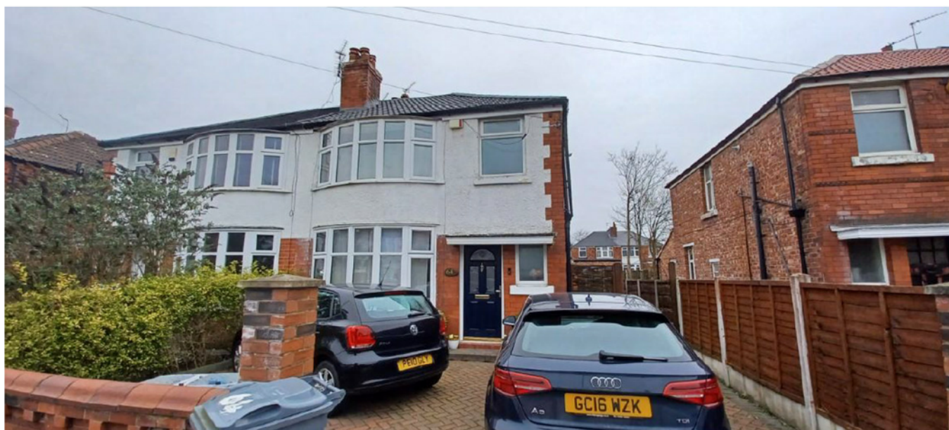
Figure 1. Principal elevation of property.
