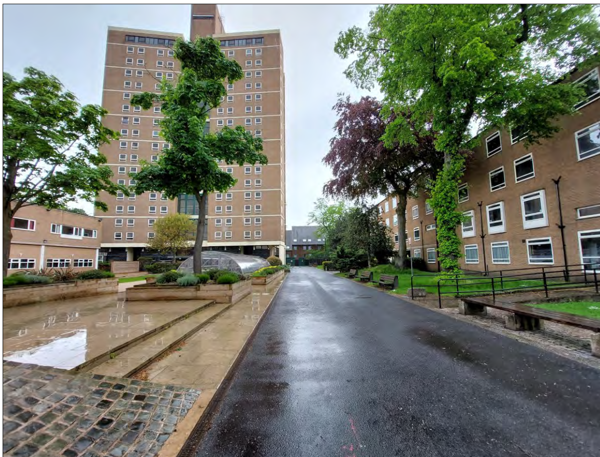
Plate 14 Photograph of the Site, showing accommodation and landscaping, facing north
