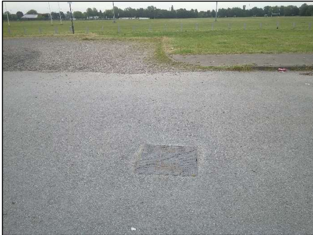
Figure 9. IC overview toward the west.
