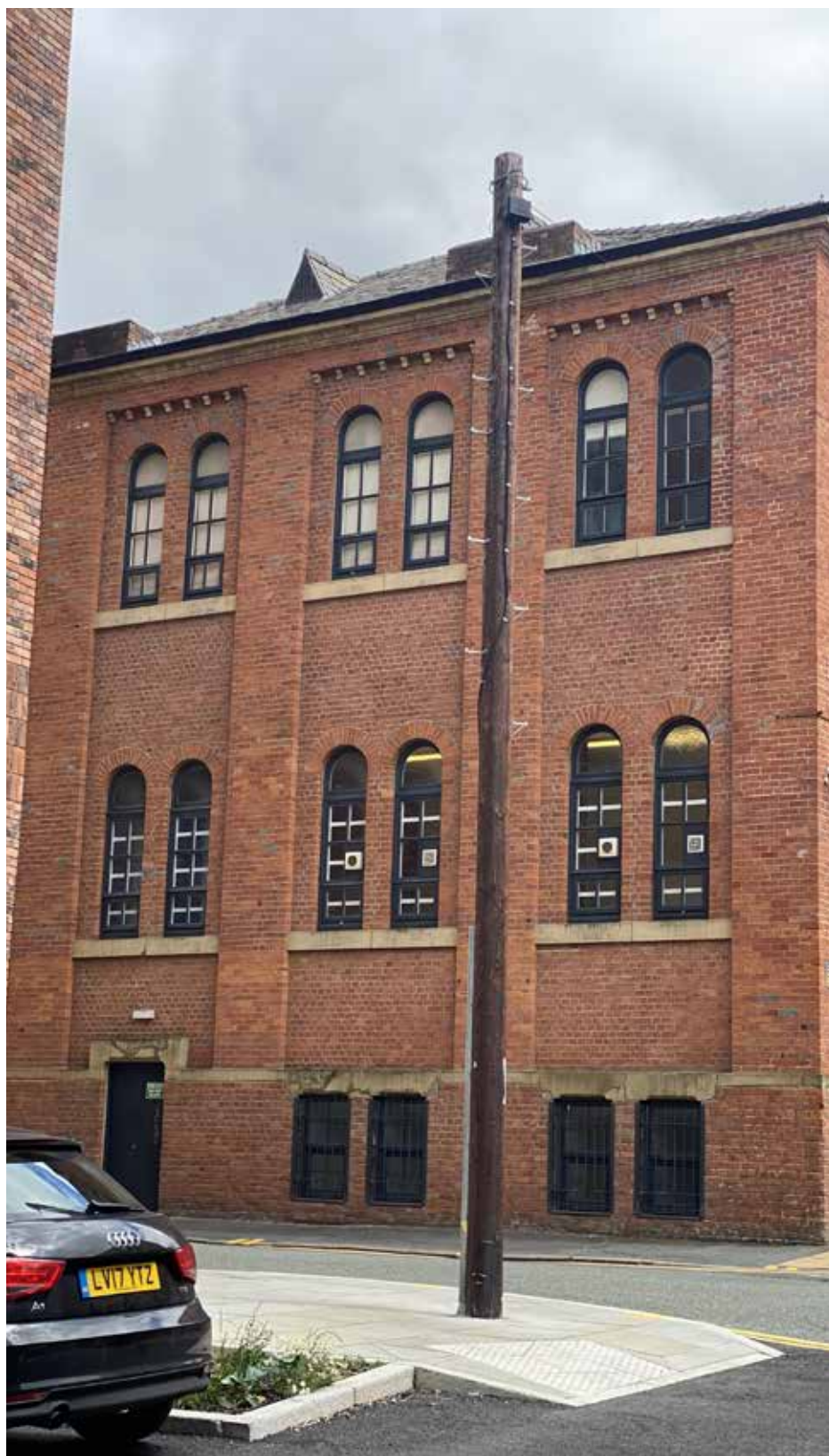
Approaching from the north (Naples Street), the red brickwork stands out, though the building is lower and less dominant in appearance.
