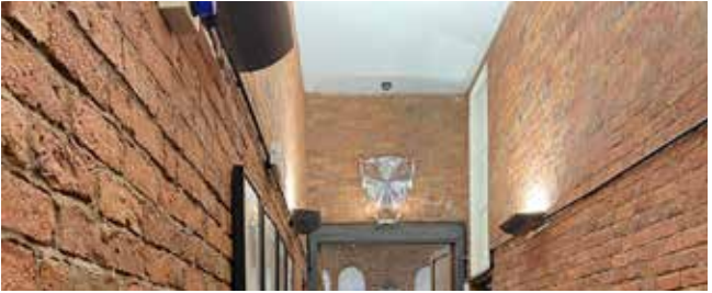
Wall mounted lights, exposed conduit and retained high ceilings
