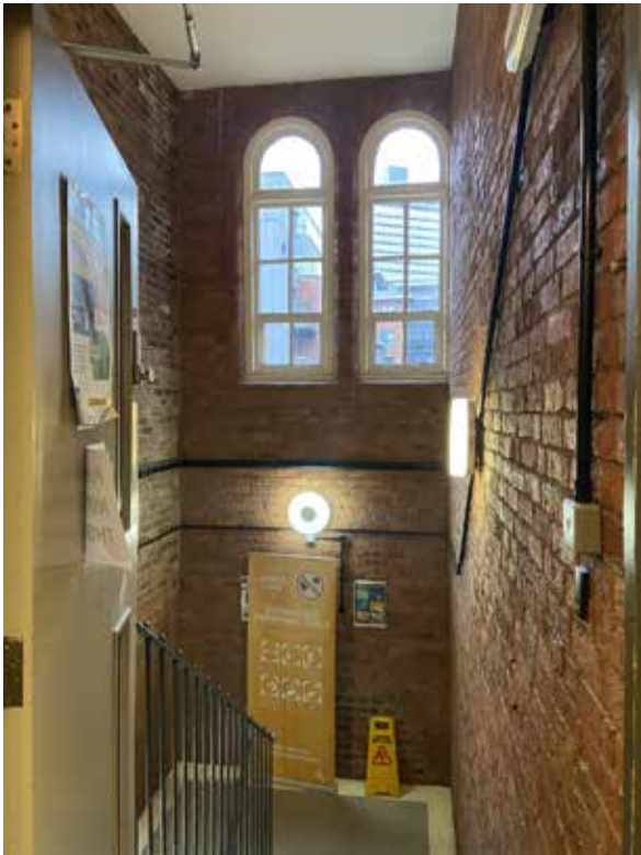
Half-landing , central staircase, modern door & brick-work. Staircase handrail detail
