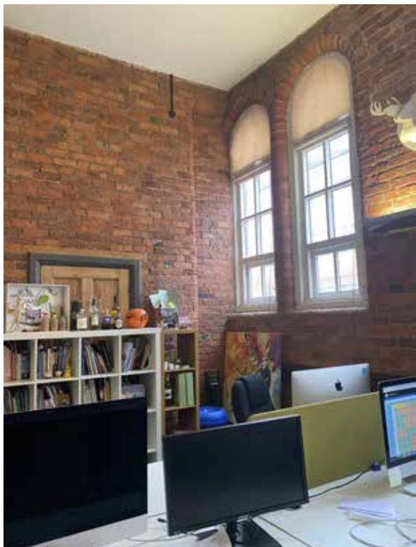
Stepped wall to window reveal
