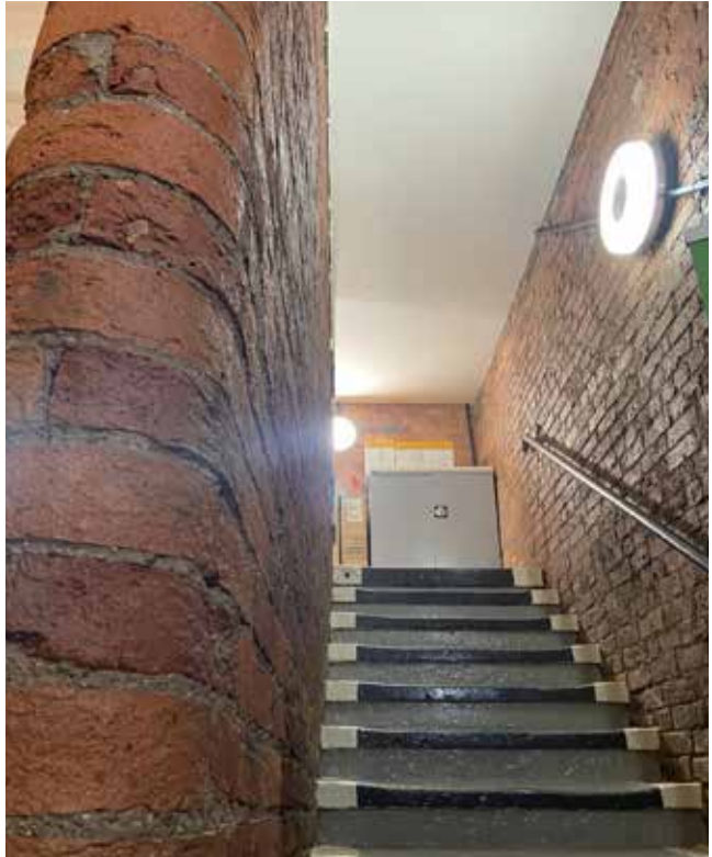
Secondary staircase, currently blocked off
