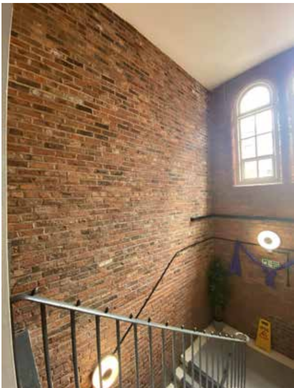
Rebuilt gable wall
