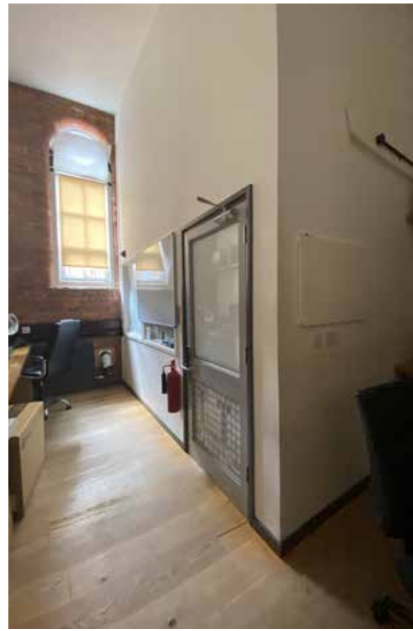
Comms room, modern infill
