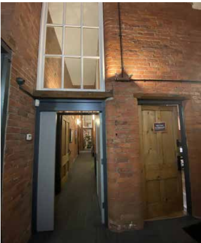
New fire doors to corridor
