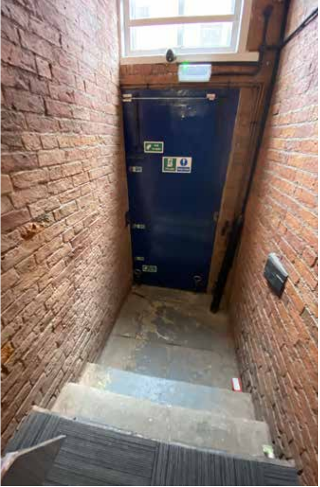
Stepped exit to school street
