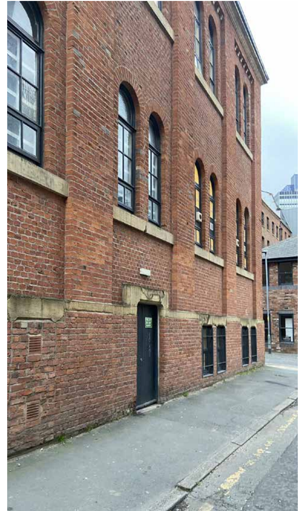
North elevation post 2010 works
