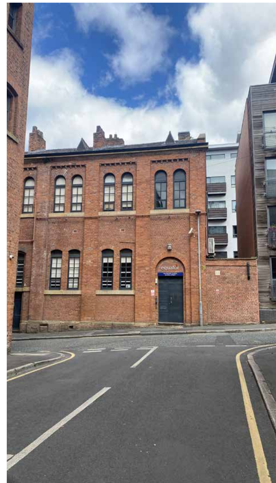
Main Entrance on School Street
