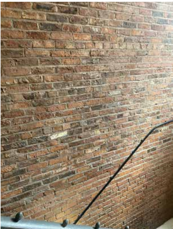
Rebuilt gable wall
