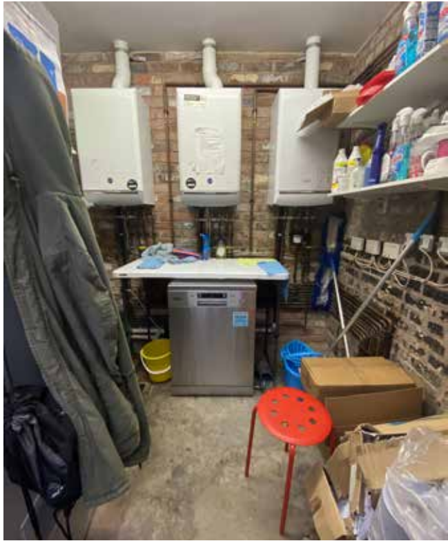
Remodelled boiler room and store
