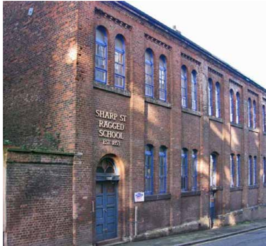
North east elevation overlooking School Street, prior to 2010 refurbishment, showing historic girls entrance.
