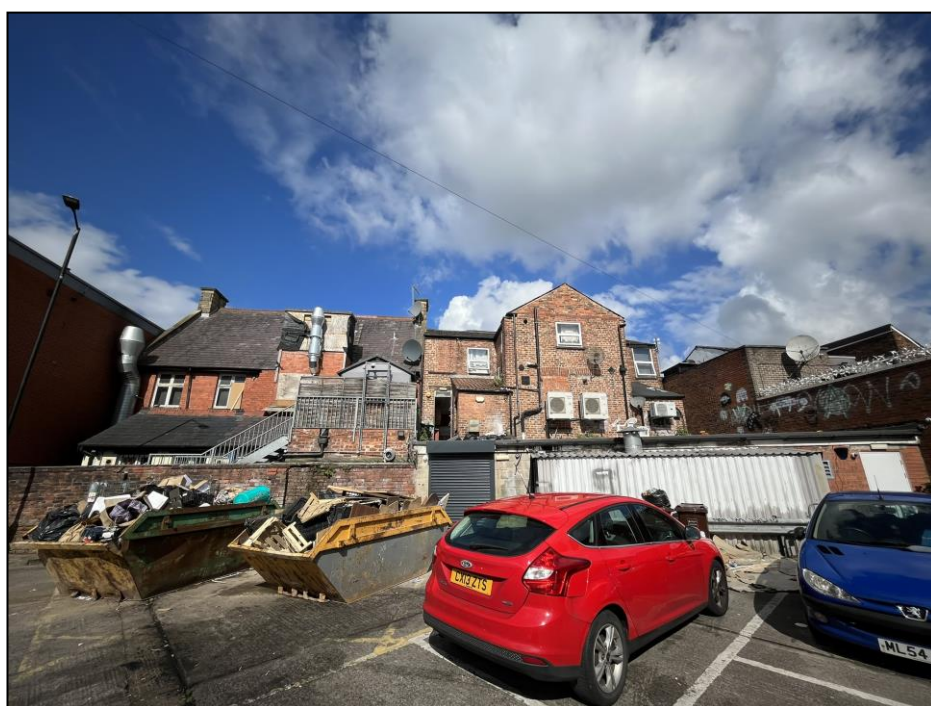
Figure 2. View from rear service yard
