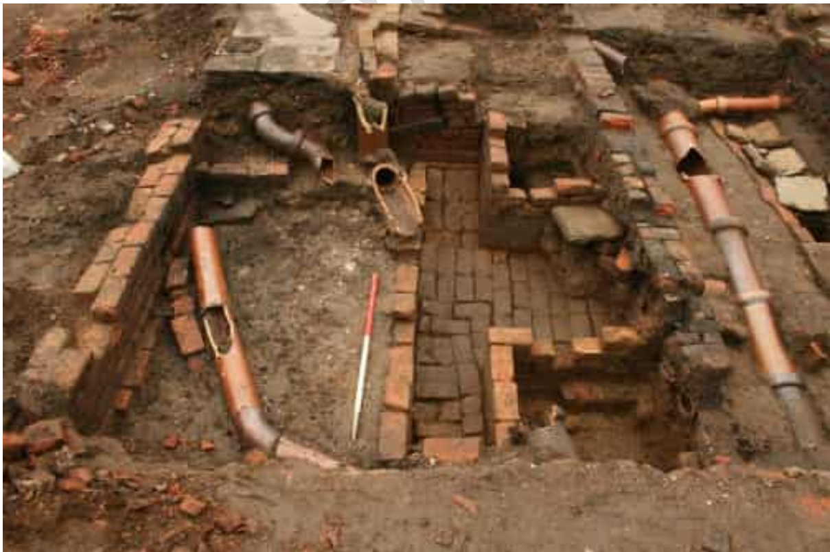
Plate 14: Remodelling of H9 yard showing later drainage [835] and earlier coal store and chute [829]
