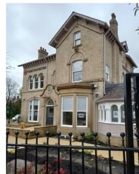
COMPLETED CONVERSION INTO OFFICES (LEFT)
