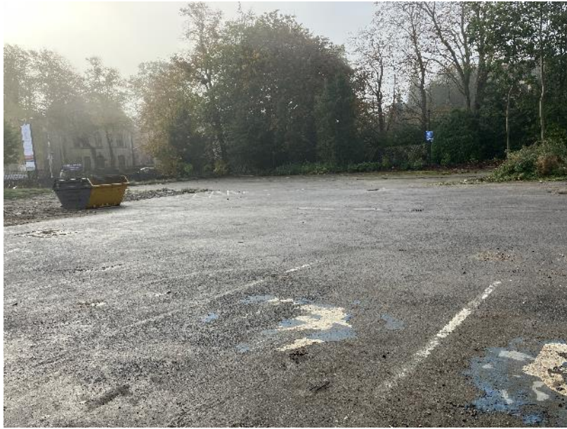
PLATE 1 SHOWING AREA OF HARDSTANDING
