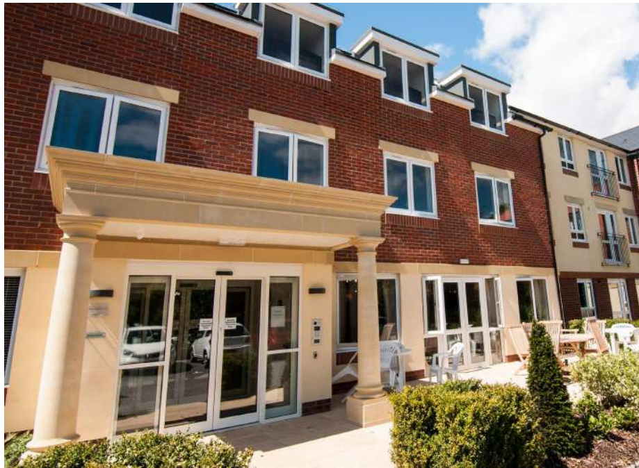
SECURE MAIN ENTRANCE FROM PARKING
