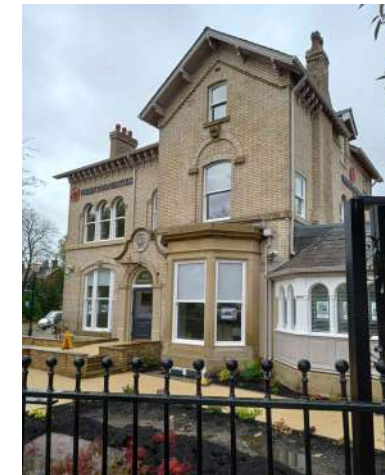
COMPLETED CONVERSION INTO OFFICES & APARTMENTS (LEFT)
