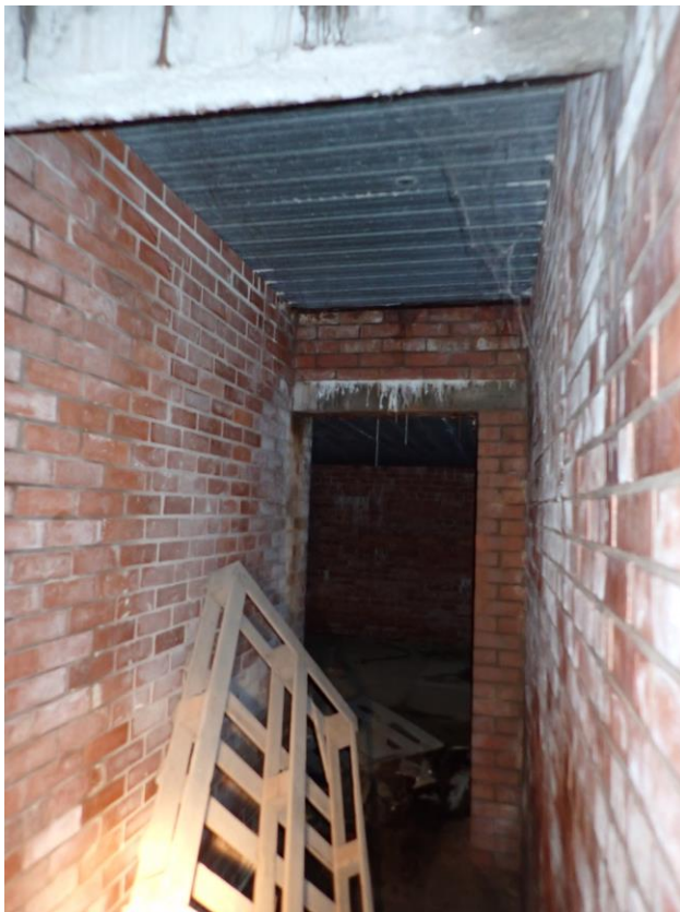
Photograph 6. A room with a metal ceiling located in the northern section of the basement.
