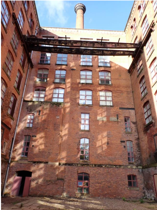
Photograph 1. The southern aspect of the building, showing an access point above the door.
