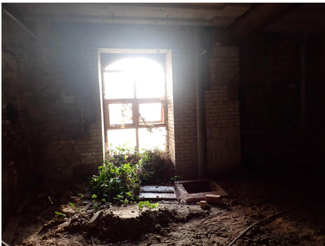
Photograph 11. A window in the southern section of the site.
