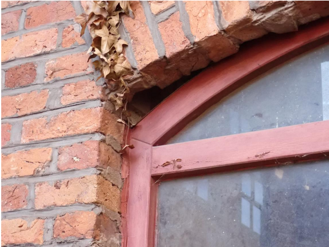
Photograph 3. Access point above a window frame on the southern aspect of the building.
