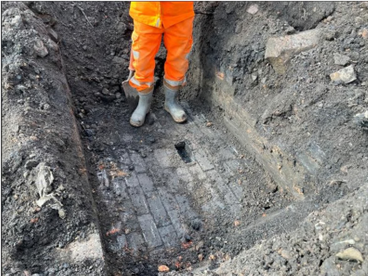
Photograph 3: CS6. Brick paved area with brick removed to allow sampling of areas of visual and olfactory contamination.
