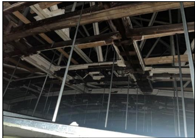
Photo1: Curved Structural Beams supporting glazed roof
