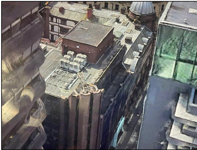
Figure 7: Aerial photo of north east rear elevation, showing proposed lift shaft location to right of rainwater downpipe (top left)
