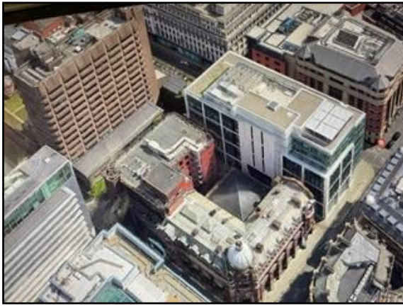
Figure 3: Aerial photo of pyramid roof over service area behind 1-3 York Street. The picture is looking north-west. The street block is bounded by York Street (bottom right), Milk Street (top) Marble Street (left) and Spring Gardens (bottom centre).
