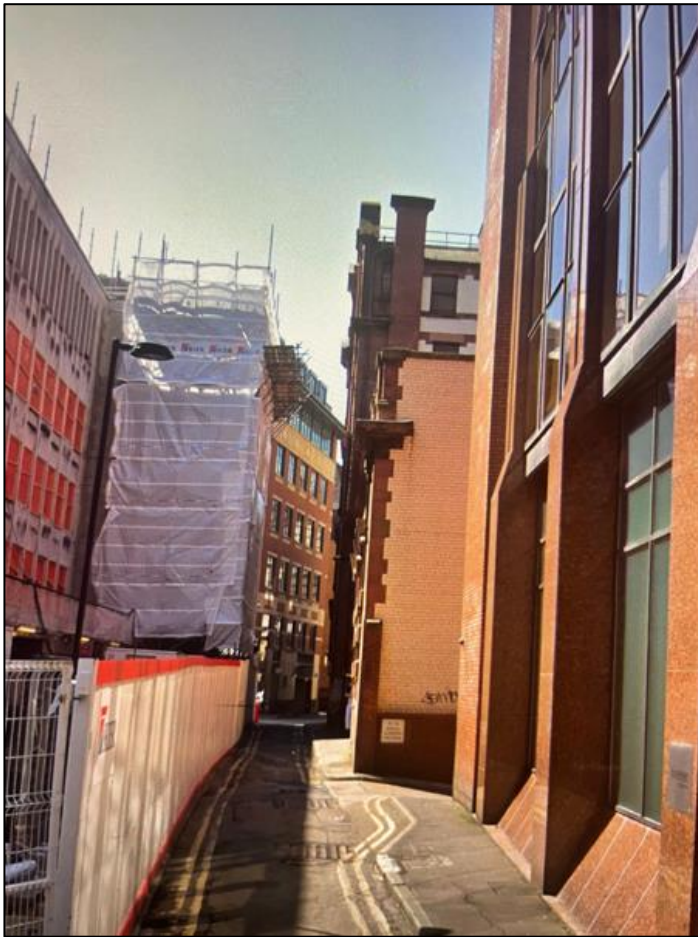
Photo 5: Viewpoint 4 Milk Street looking south from Marble Street. New development in progress on left, service area to 1-3 York Street centre, 19 Spring Gardens on right.
