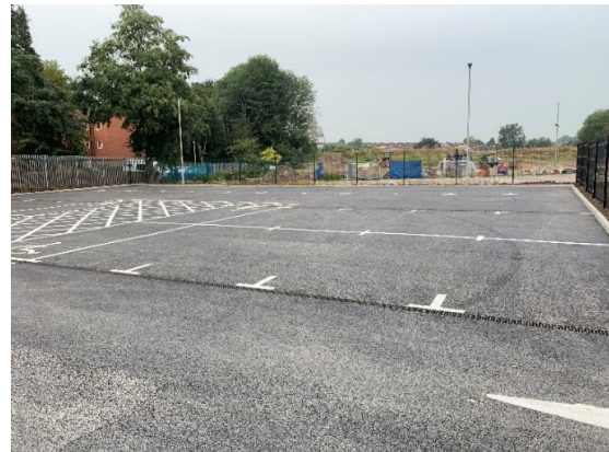
Photo 8 – Macro between 2 drainage channels
