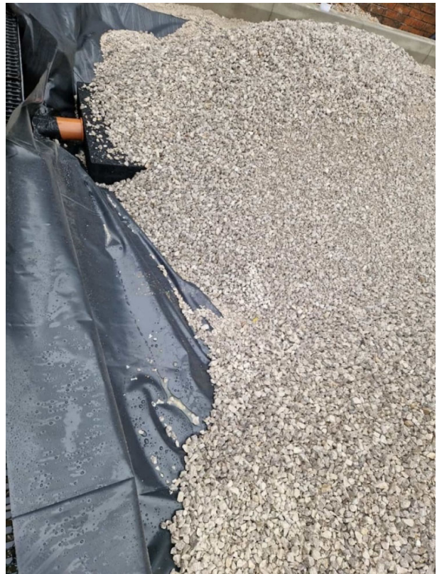
Photo 4 - Macro construction. Clean stone
