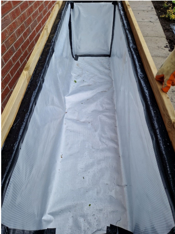
Photo 11 -Planter before pipework and filling
