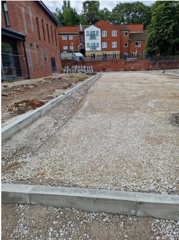
Photo 1 – Formation Level. Looking towards SE
