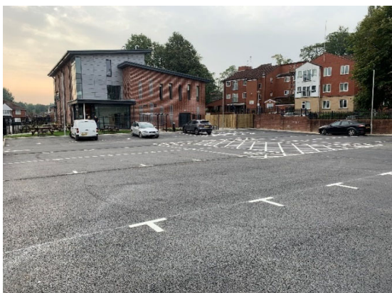
Photo 9 - Macro between 2 drainage channels
