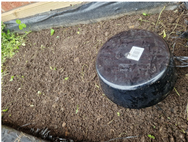
Photo 13 -Overflow pipe reduced in height. Now set 100mm below top of planter 1.
