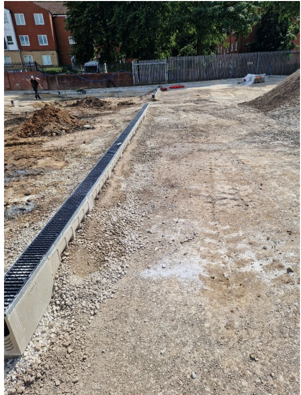
Photo 2 – Formation level. Macro on right
