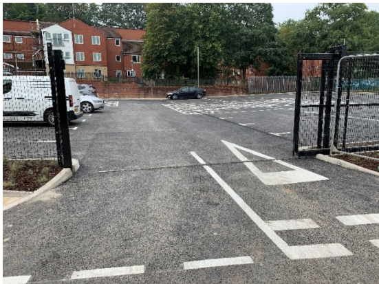
Photo 7 – Final car park entrance
