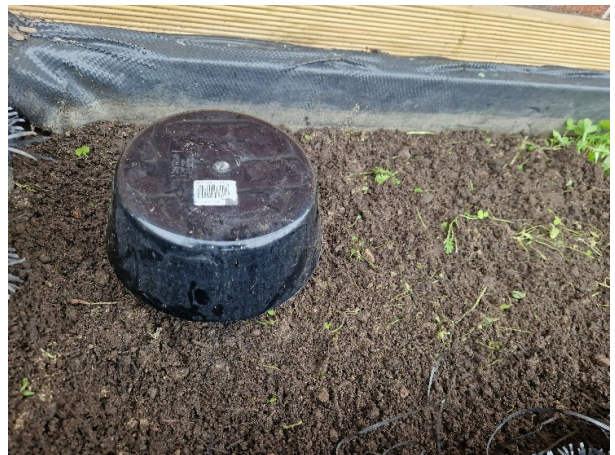
Photo 14 - Overflow pipe reduced in height. Now set 100mm below top of planter 2.
