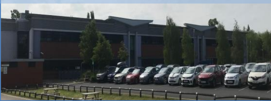
A view of the western elevation of Withington Community Hospital and adjacent car park from Nell Lane
