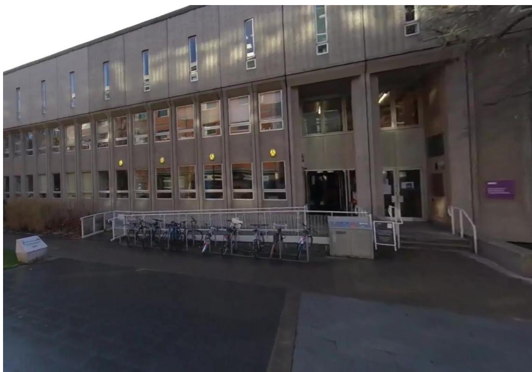
Figure 6.6: Existing entrance ramp proposed to be removed
