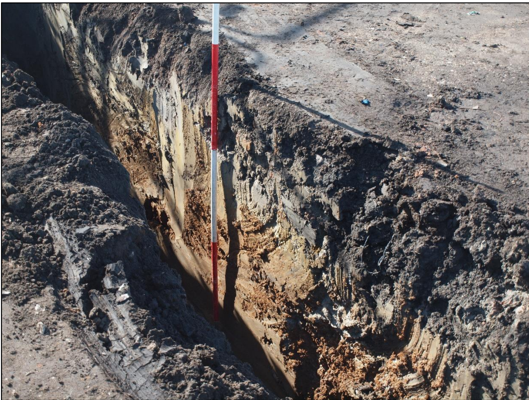
Plate 14: Section showing clay (03) close to surface
