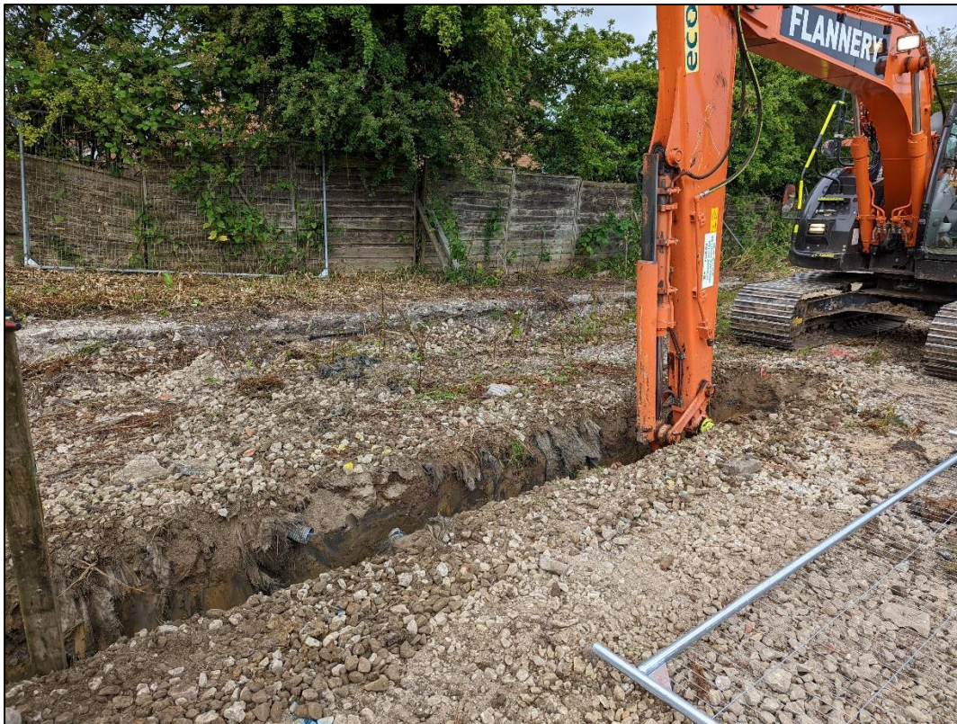
Plate 9: Excavation of plots 38 & 39
