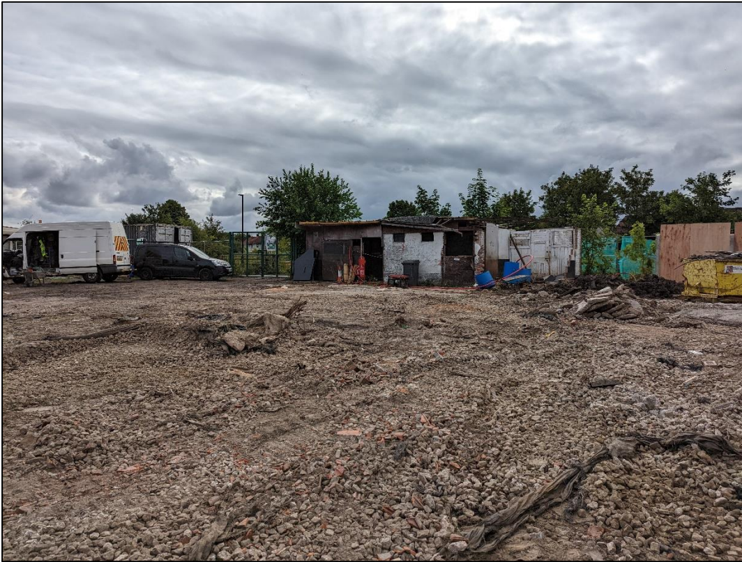
Plate 1: Site prior to excavation
