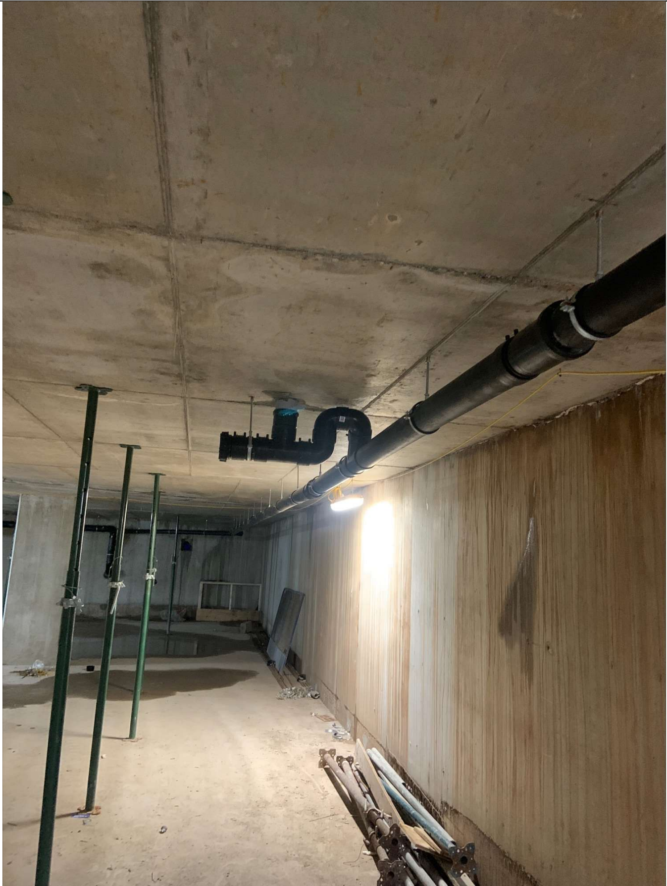
Photo 18 – Blue Roof Attenuation Crate Installation 09.02.23 viewed from Site Cabins looking West
