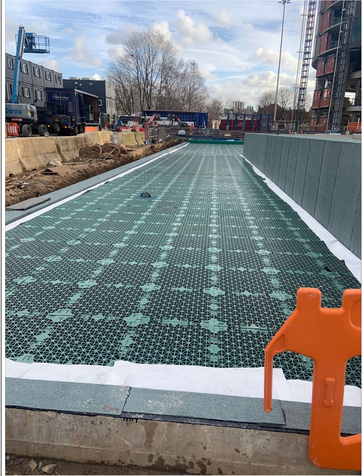
Photo 6 – Blue Roof Attenuation Crate Installation 09.02.23 viewed from ground level looking north
