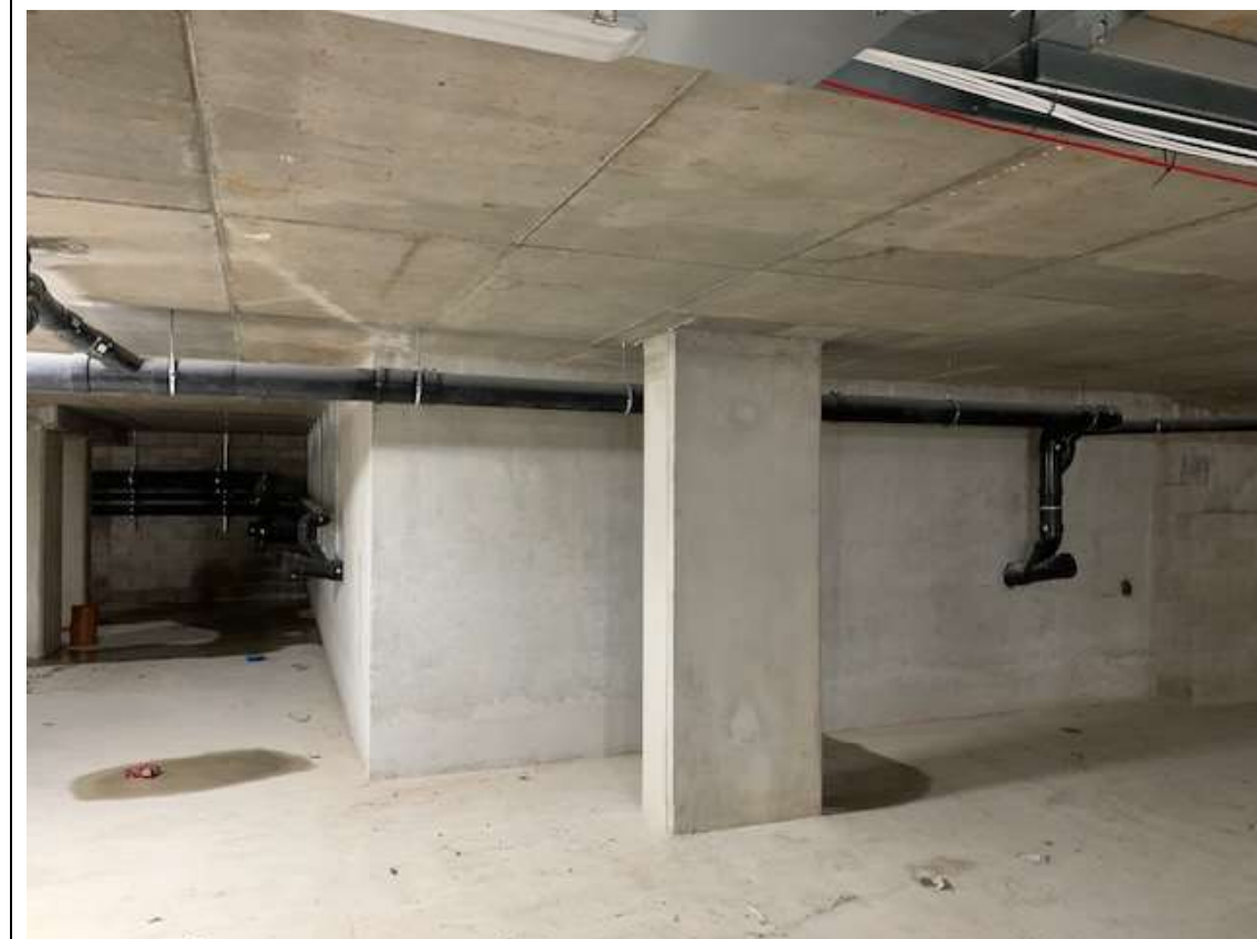
Photo 16 & 16a – B1 Level Underslung Drainage From Blue Roof Attenuation Crate To Silvercroft St Manhole
