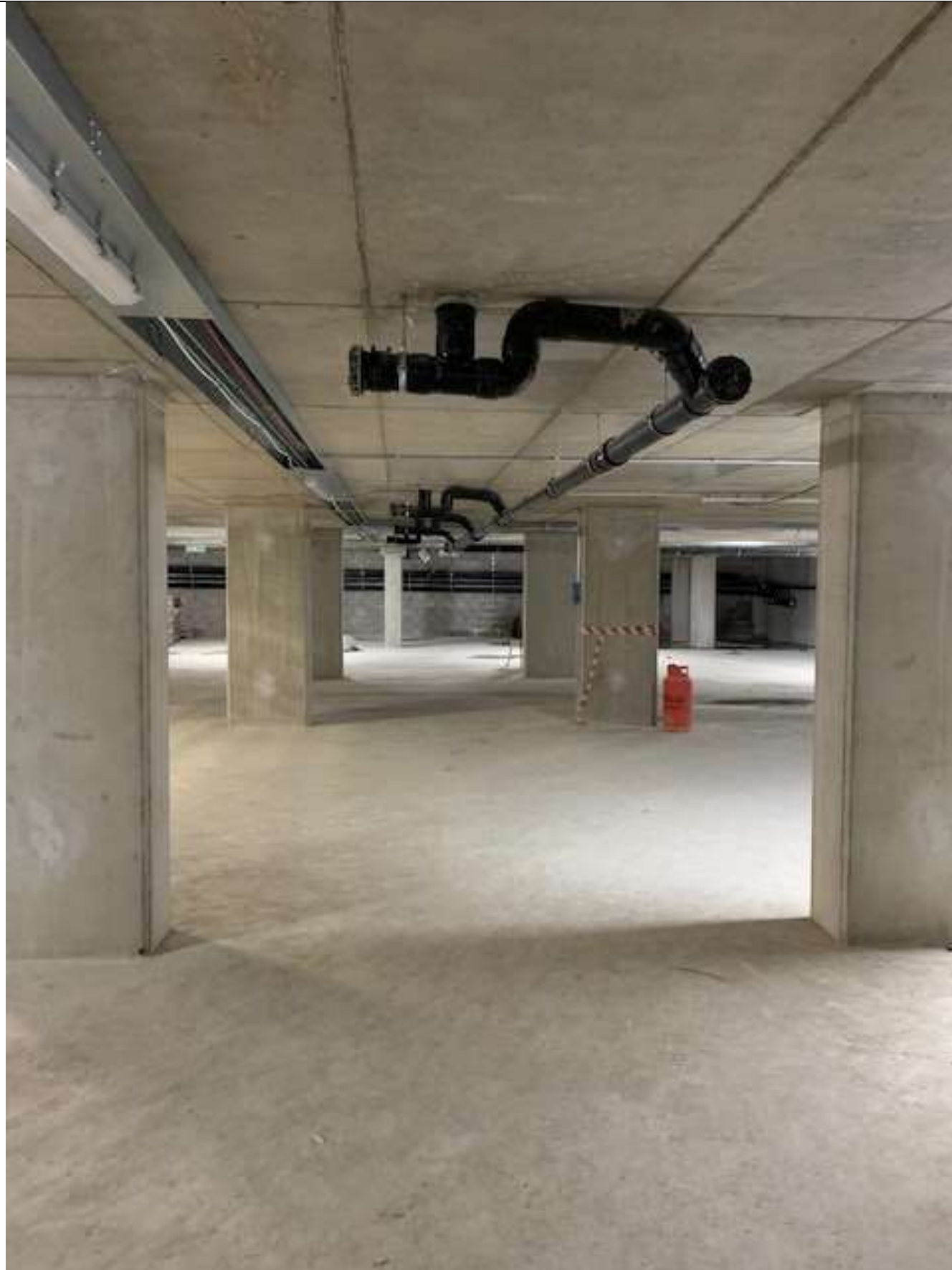
Photo 15 – B1 Level Underslung Drainage From Blue Roof Attenuation Crate To Silvercroft St Manhole
