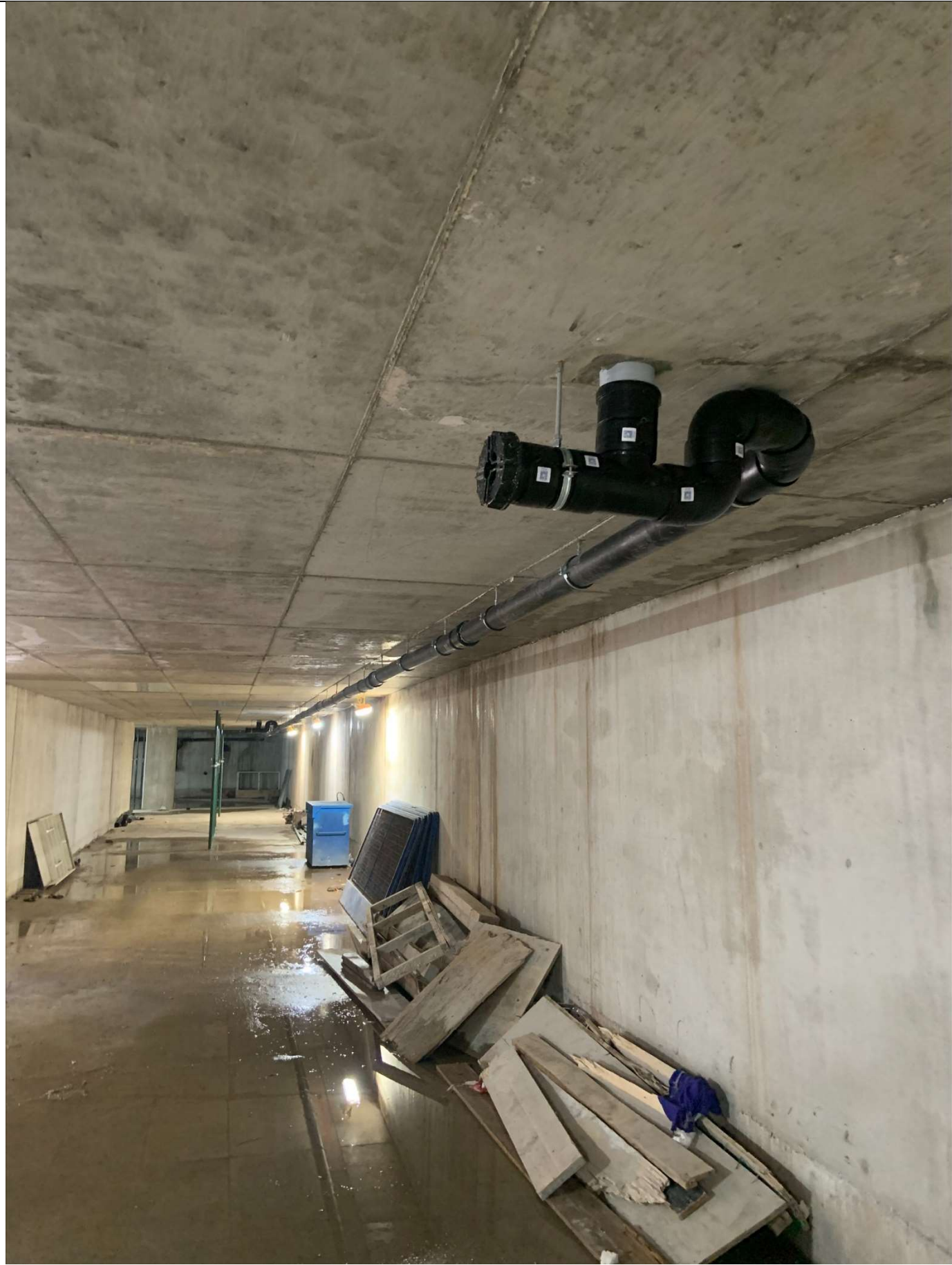
Photo 17 – B1 Level Underslung Drainage From Blue Roof Attenuation Crate To Silvercroft St Manhole
