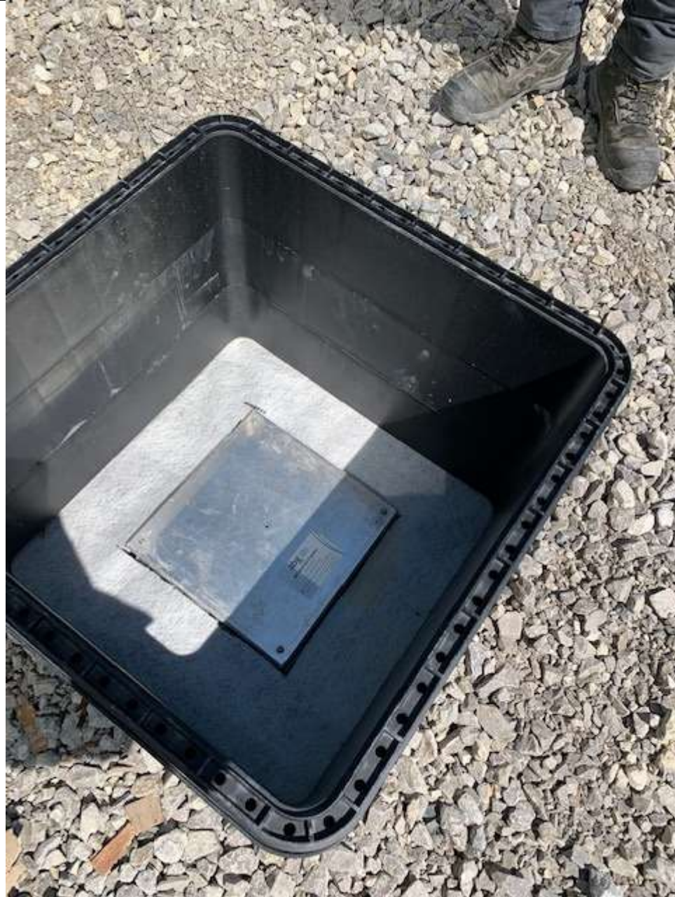
Typical Blueroof Gully chamber once complete (except lid and final finishes)
