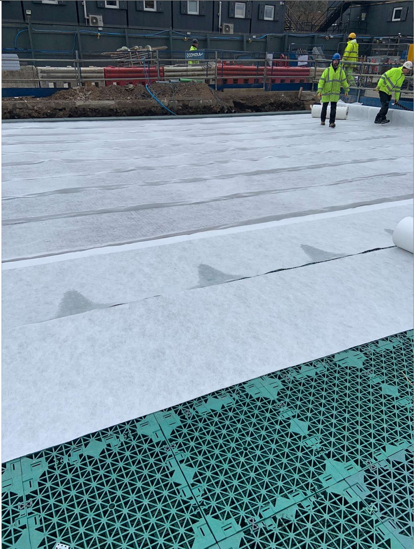
Photo 8 – Blue Roof Attenuation Crate Installation 28.03.23 viewed from ground level looking east
