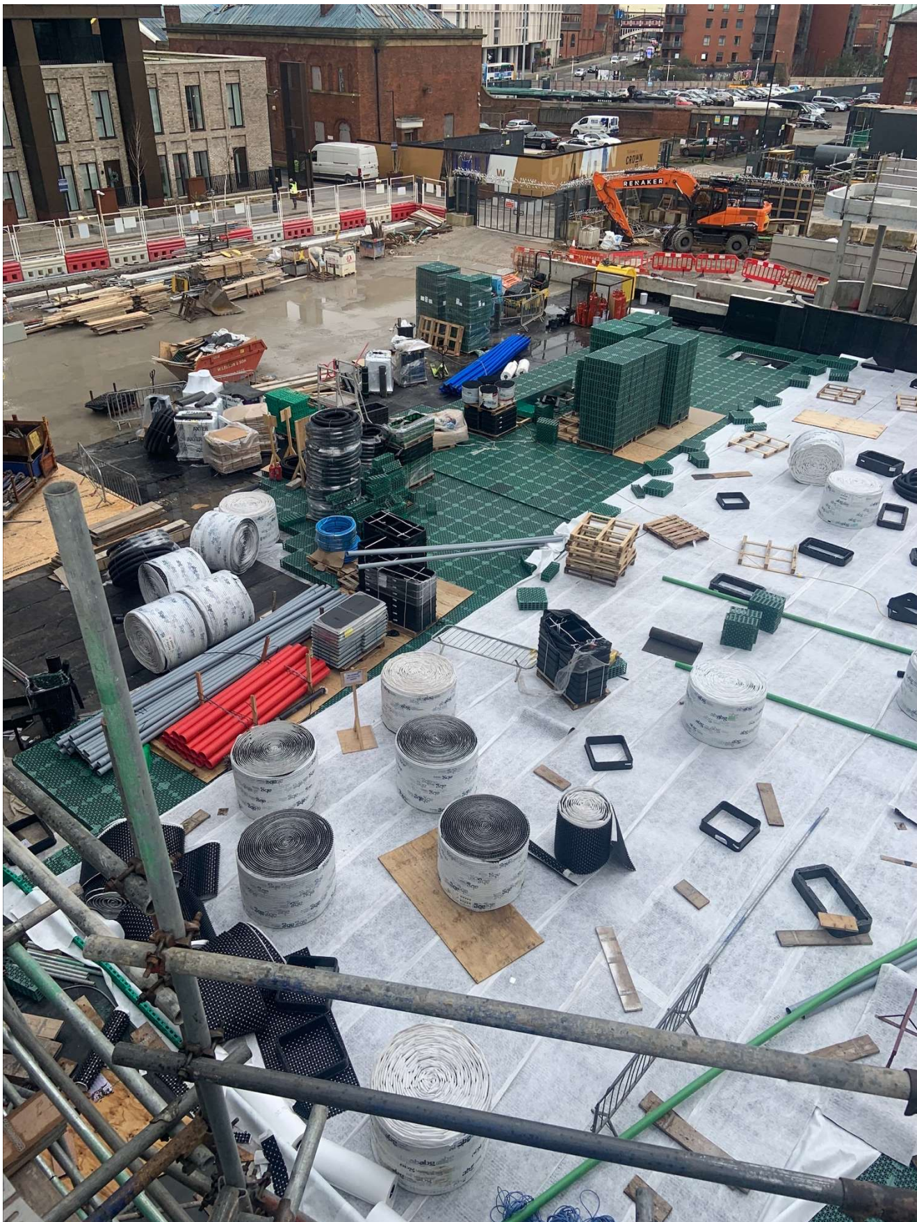
Photo 8 – Blue Roof ducting and stone Installation 29.03.23 Viewed from C5 Level 2
