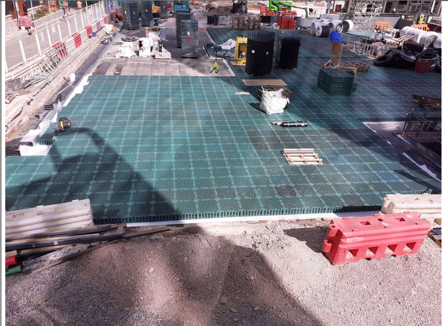
Photo 12 – Blue Roof Attenuation crate Installation 25.04.23 Viewed from School
