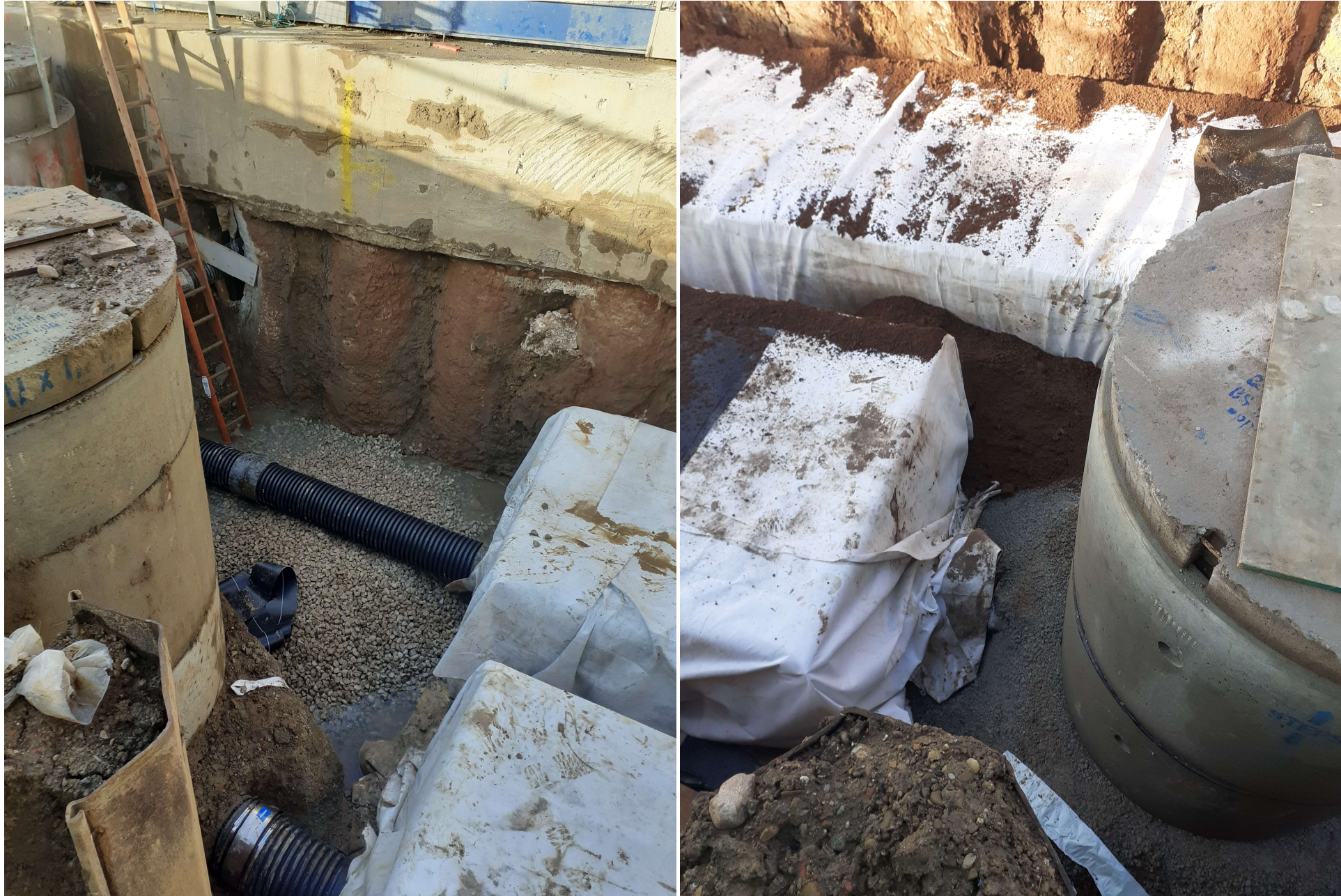
Attenuation Tanks and pipe connections complete ready for backfill
