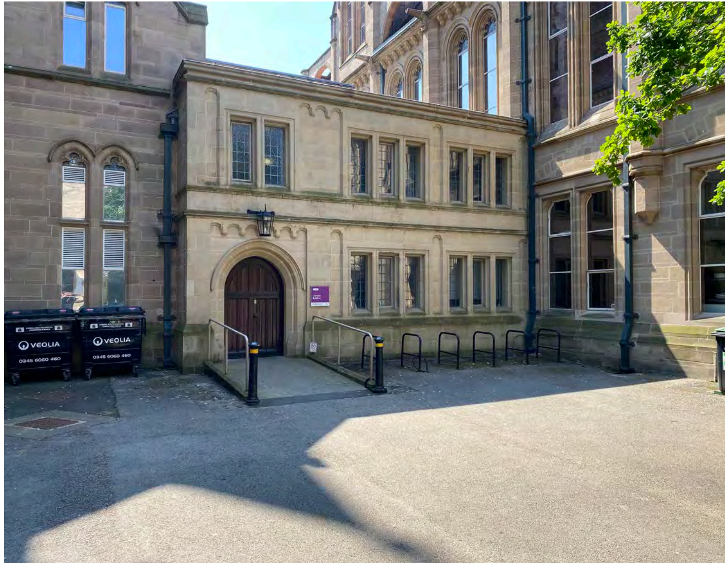
Existing Christie access / servicing space
