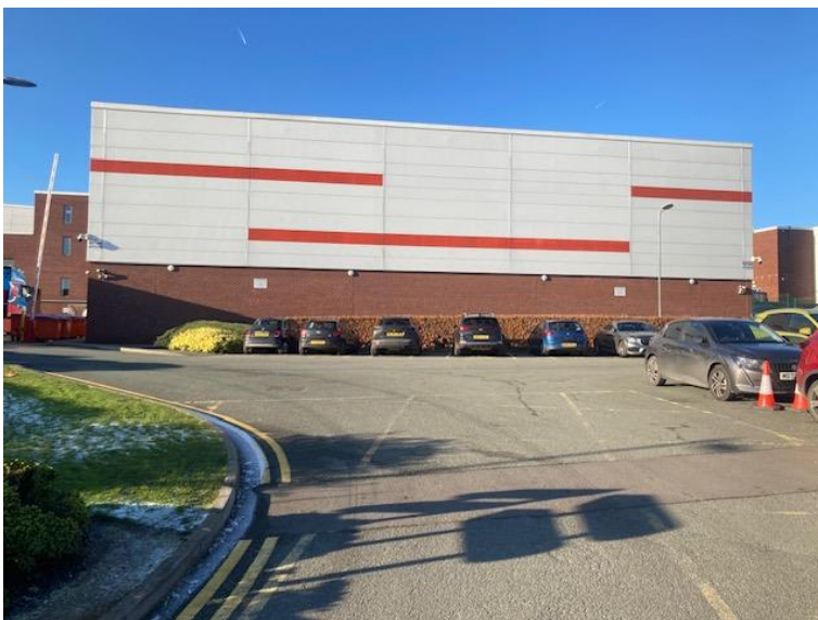
View of the disable parking spaces adjoining the existing building proposed to be extended
