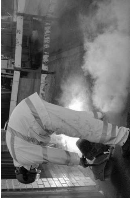
Figure 1 Common tasks like cutting can create very high dust levels
