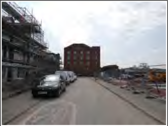
Looking South along Newton Street Towards Newton Silk Mill, with East Boundary to Proposal Site on Right
