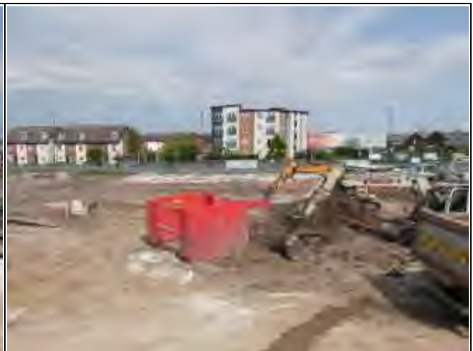
Looking North Across West Side of Proposal Site
