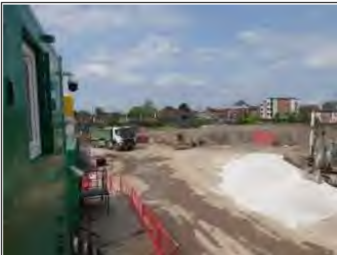
Looking Northwest Across West Side of Proposal Site
