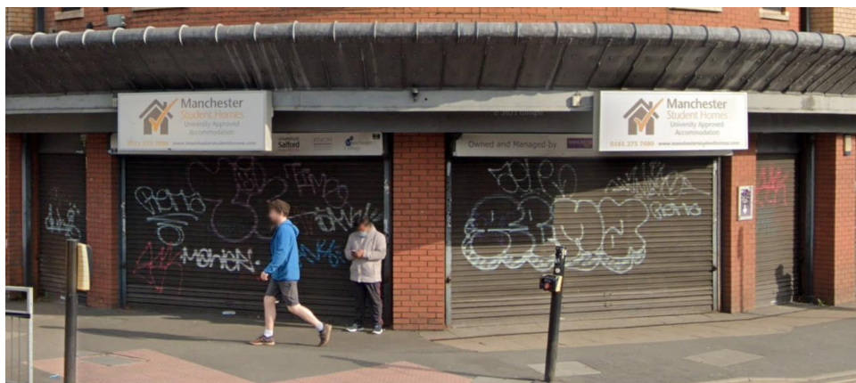
Existing Frontage of Units 1-3
