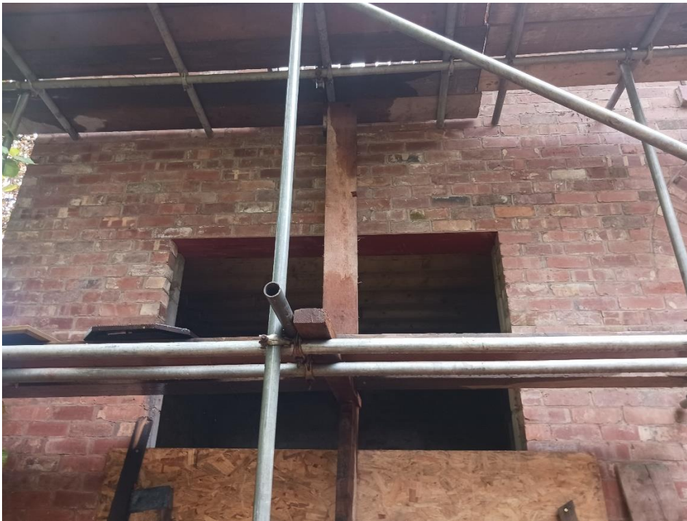
Ground floor window bay
