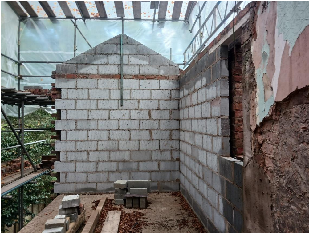
Internal view of outrigger at first floor
