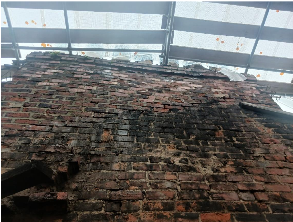
View of chimneys of 4 Park Avenue and party wall
