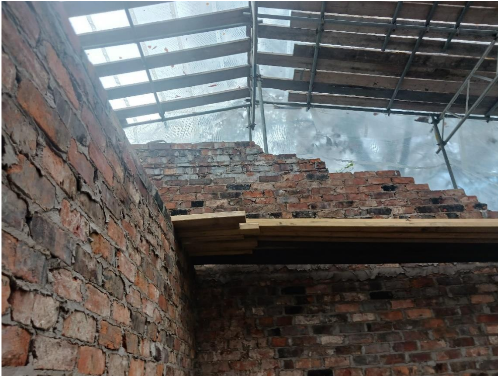
View to end gable wall and chimney
