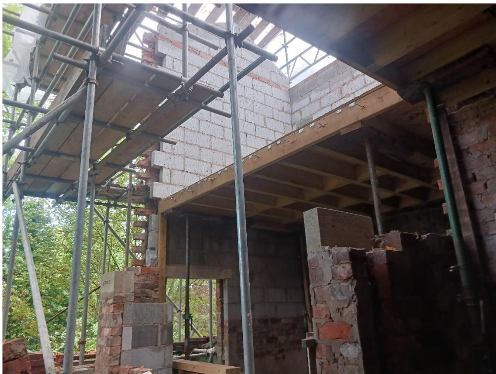
View from within property looking towards outrigger
