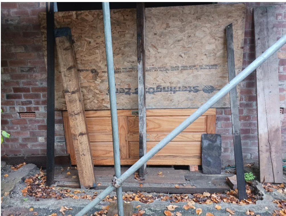
Ground floor window bay
