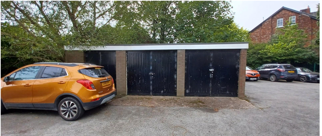
Figure 6. Garage (to be demolished).
