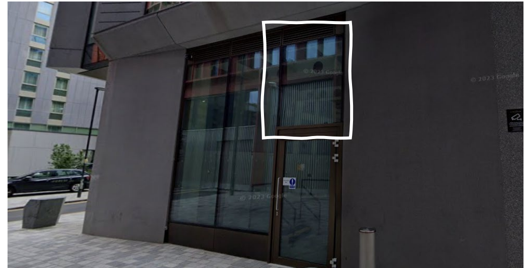
Existing arrangement - two glazed panels (Google street view)
