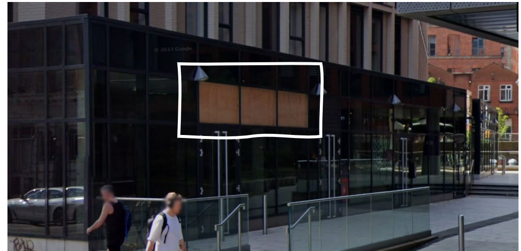
Existing arrangement (Google street view)
