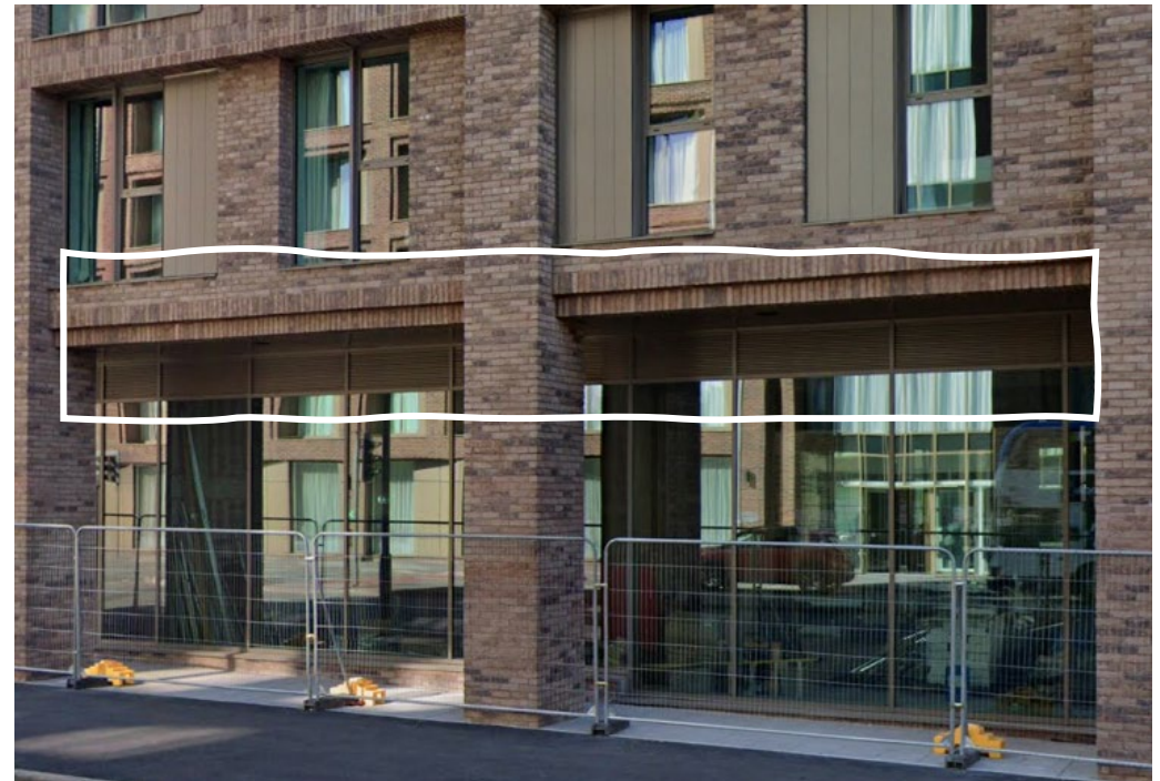
1 – Louvres above windows at ground floor (Google street view)
