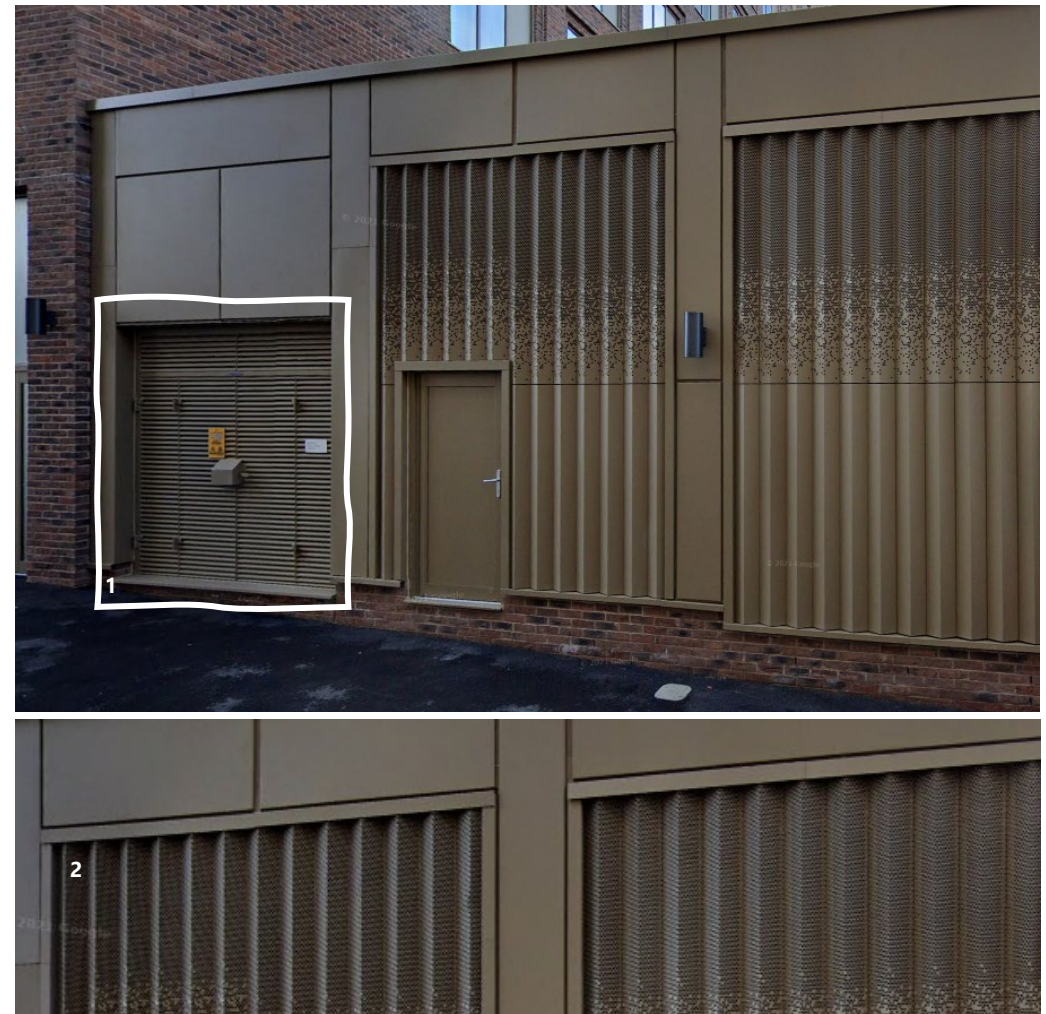
1 & 2 – Louvres and perforated cladding to provide ventilation (Google street view)
