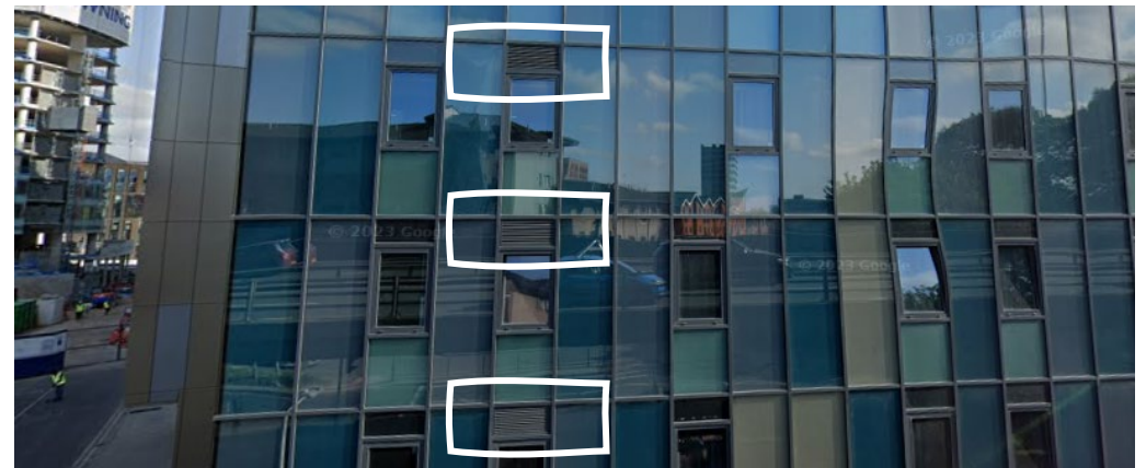
Block 2 – louvres above windows on south elevation (image from Google street view from Ring Road)
