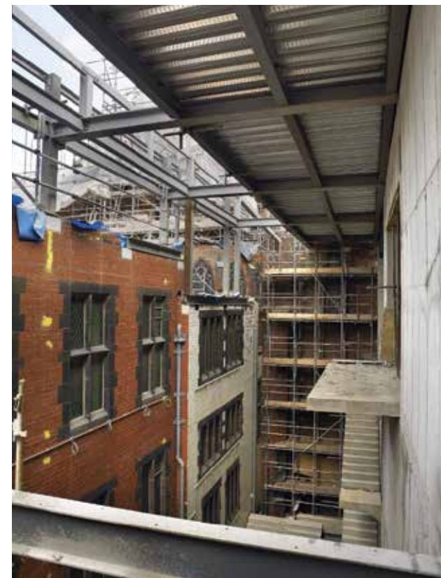
Construction of the 2007 building, 2006
