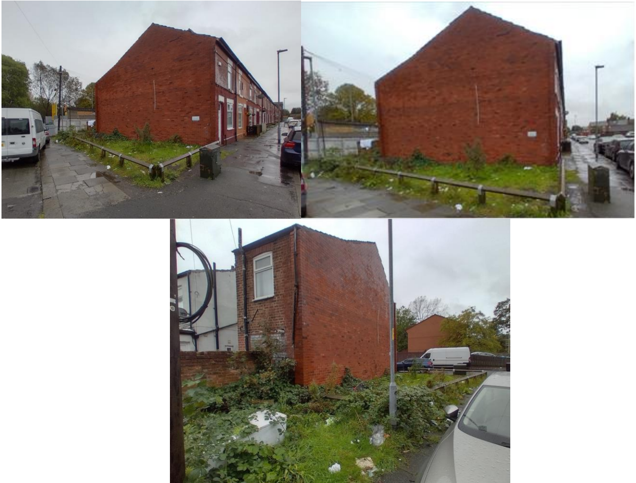
Fig.1 – Views of the application site.
