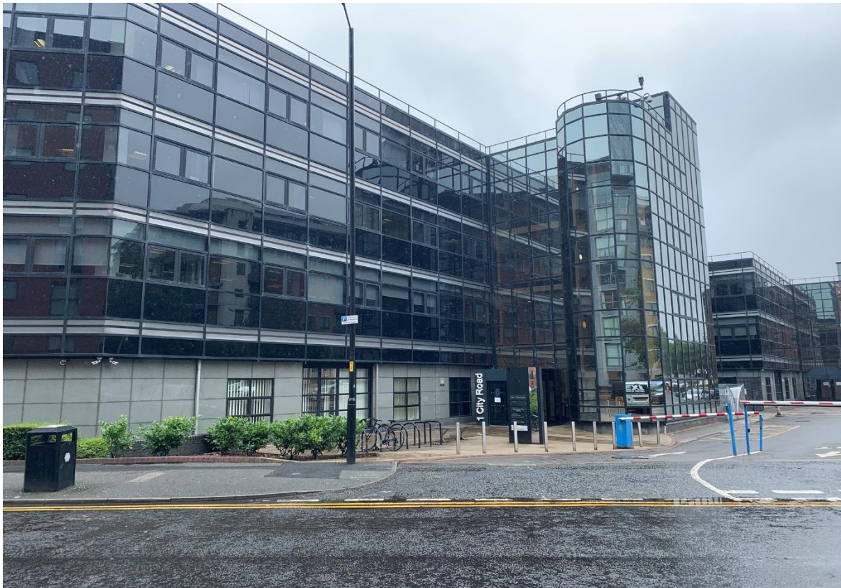
Plate 1 – No 1 City Road Office Development in East of Site Looking South
