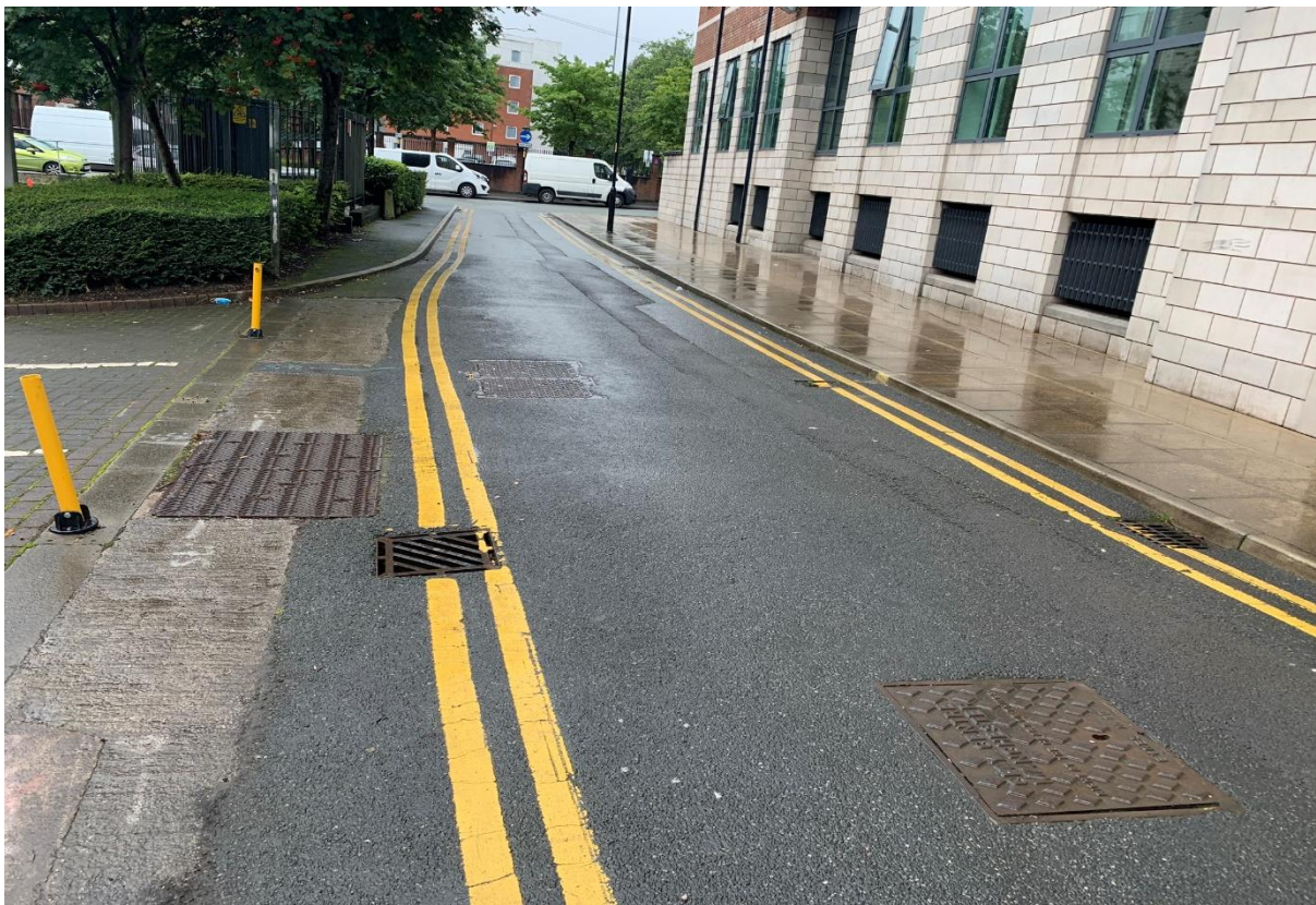
Plate 10 – Western Boundary Looking South
