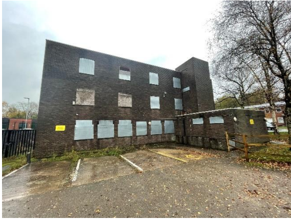
Photograph 5 – First building and associated car park
