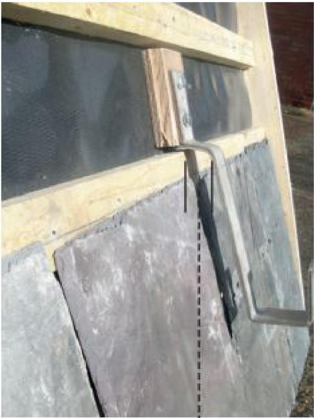
Slate roof showing 30mm clearance
