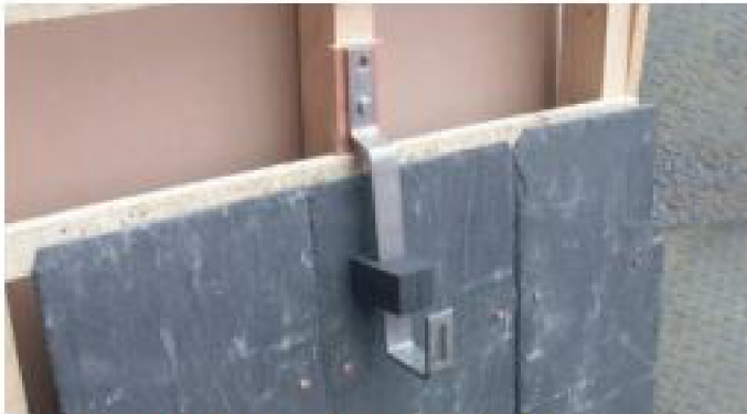
Step 1: Fix foam to bracket drop.
