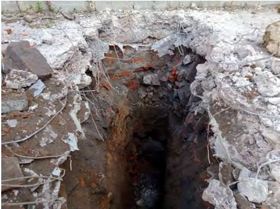
Photograph 5: View of brick retaining wall exposed in TP105.
