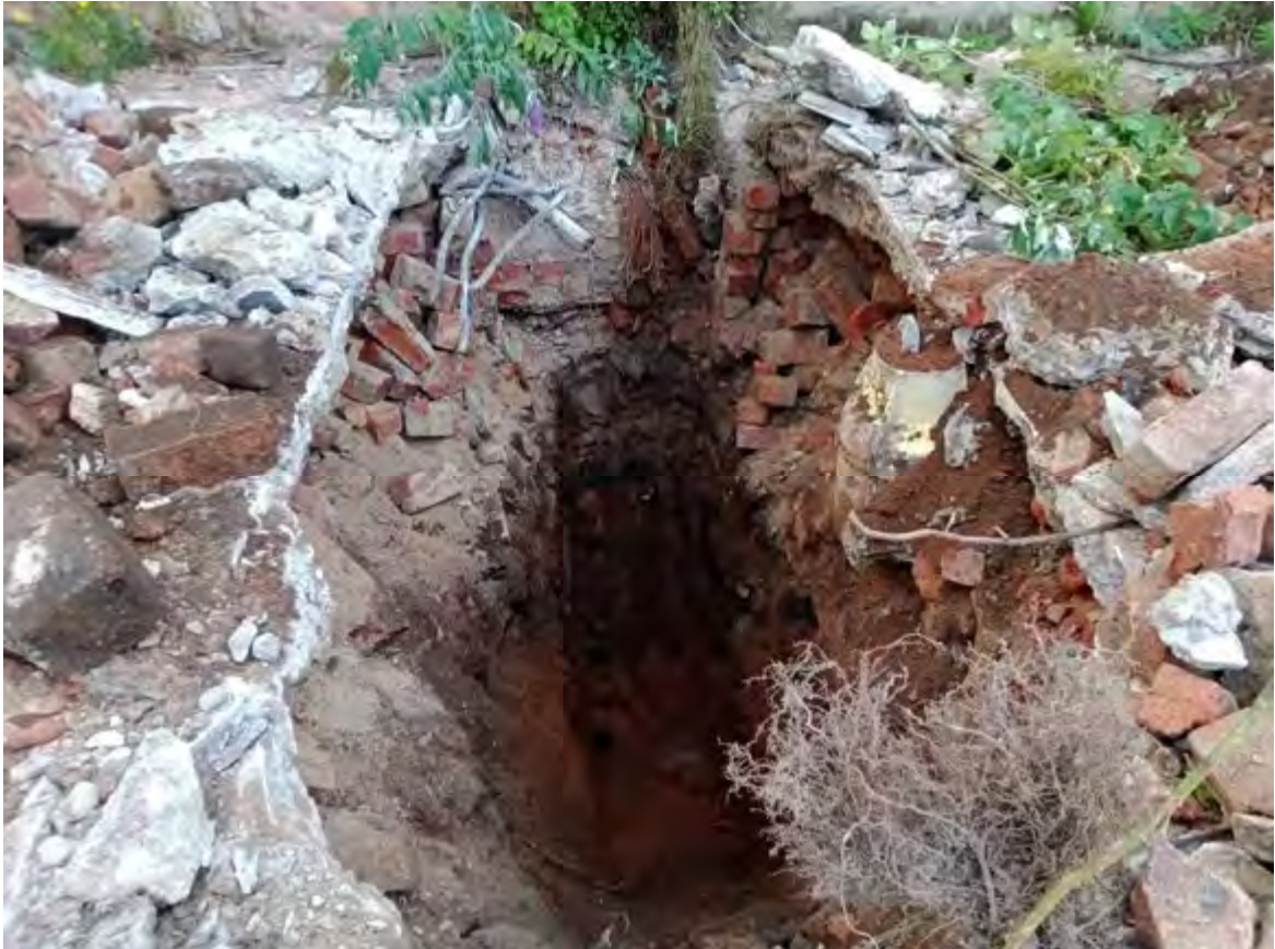
Photograph 4: View of brick retaining wall exposed in TP103.
