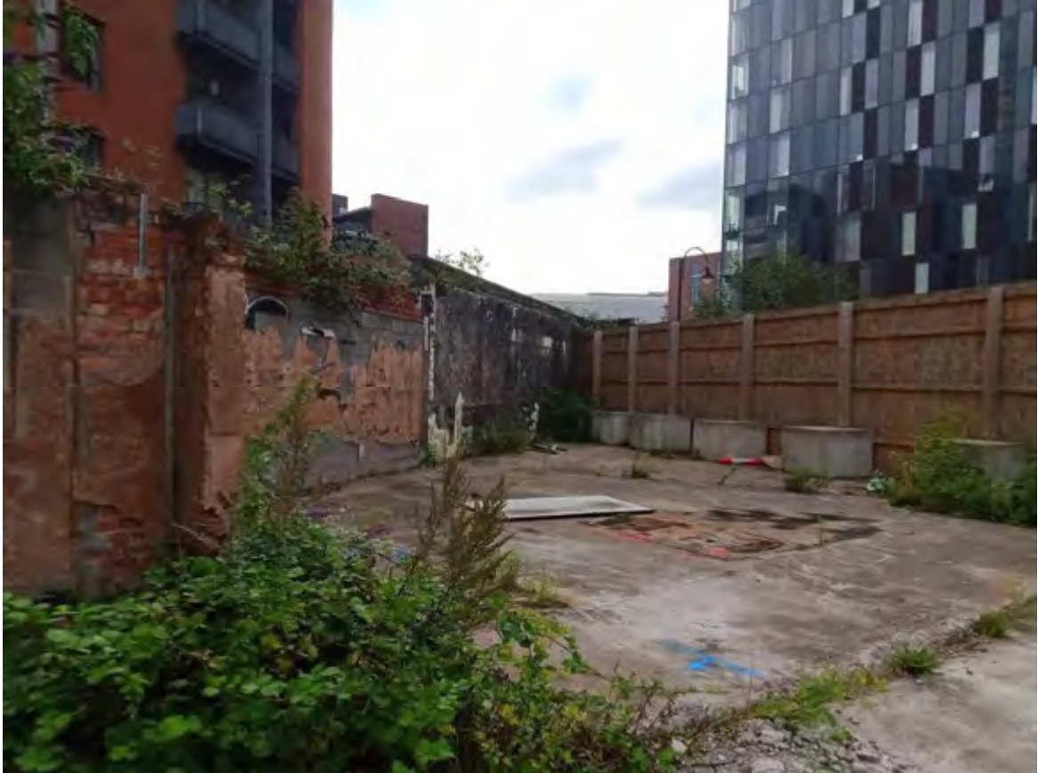
Photograph 3: View of southeast corner, showing derelict manholes.
