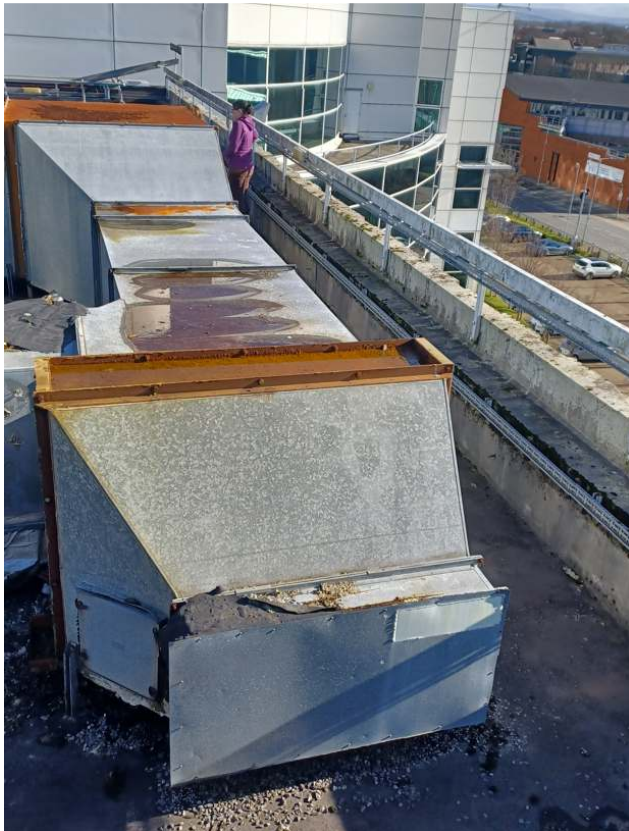
Existing roof view from south west to east
