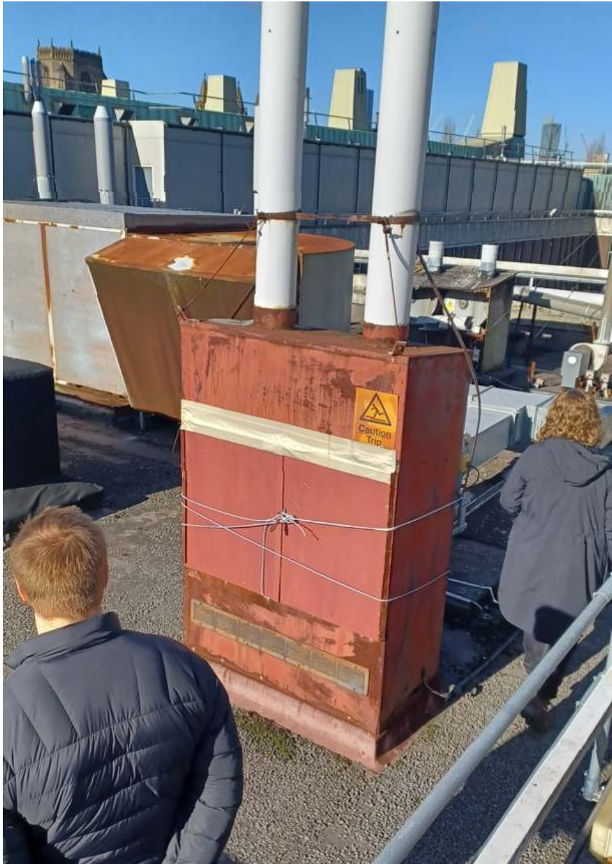
Existing roof view from south west to north
