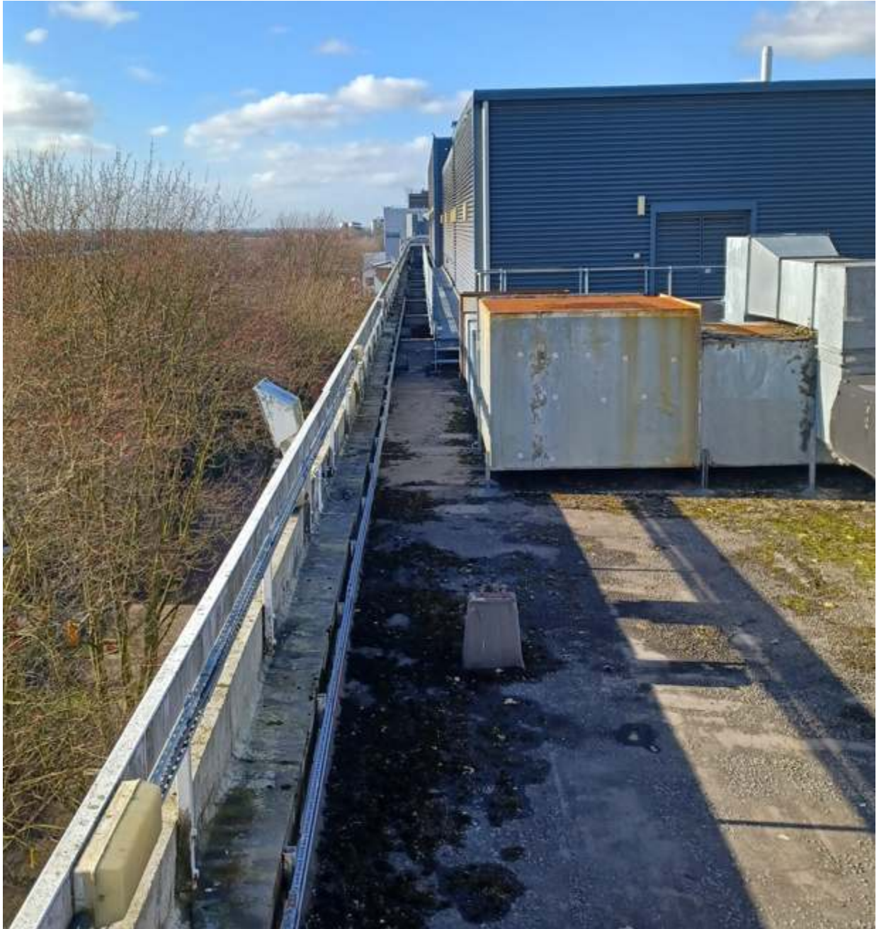
Existing roof view from south west to east
