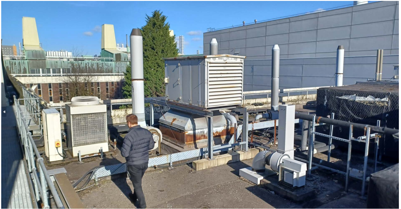
Existing roof view from south west to north
