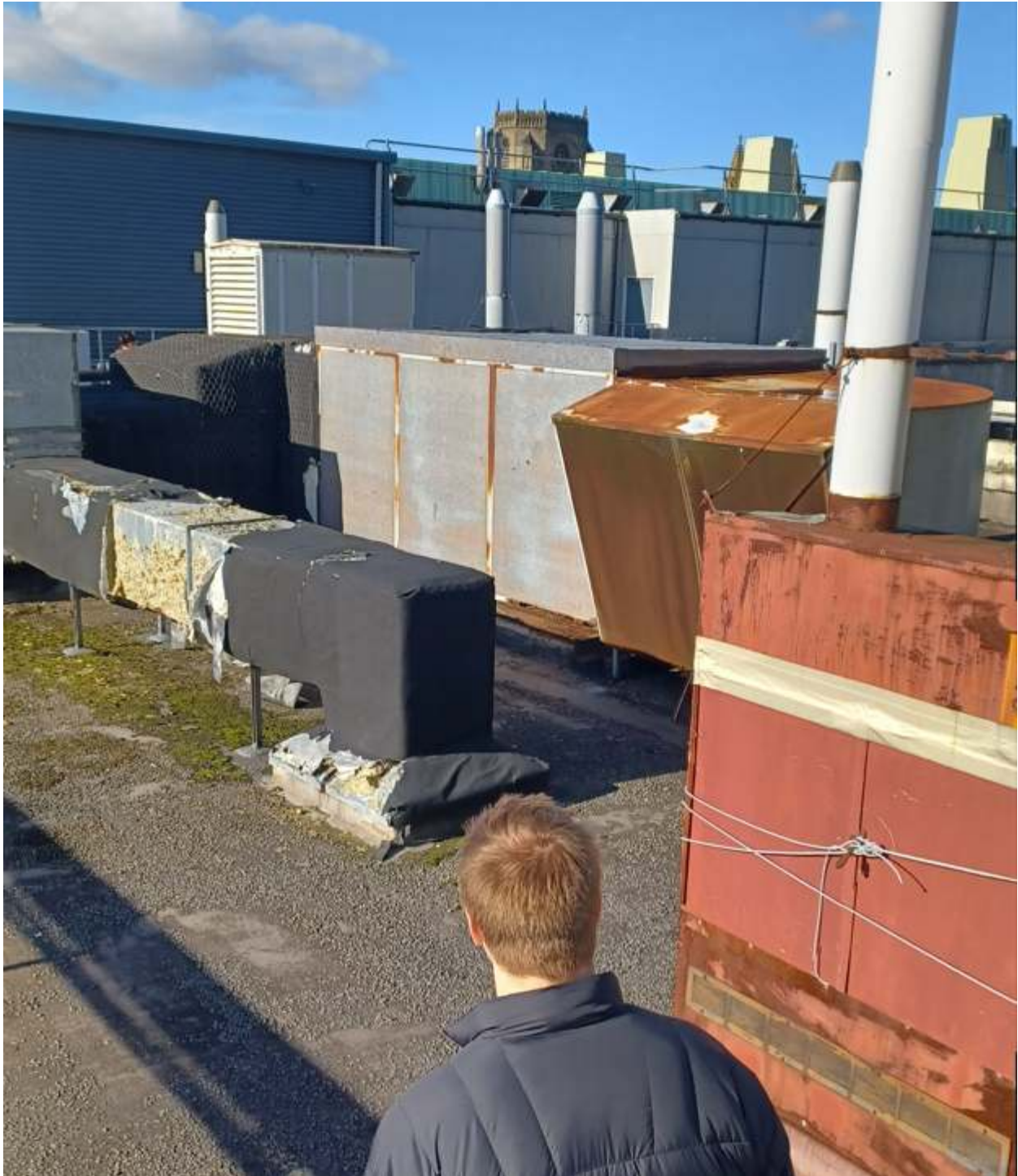
Existing roof view from south west to north east
