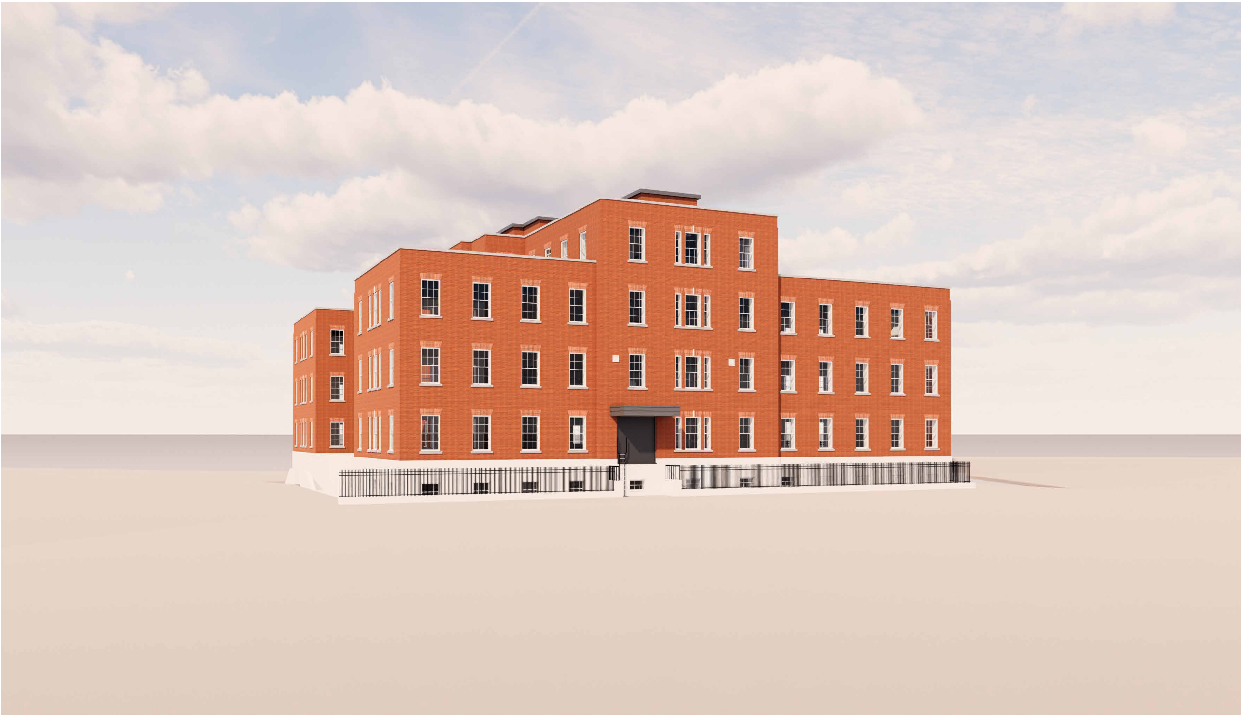
06 - Existing view of the Zochonis Building from Dover Street
