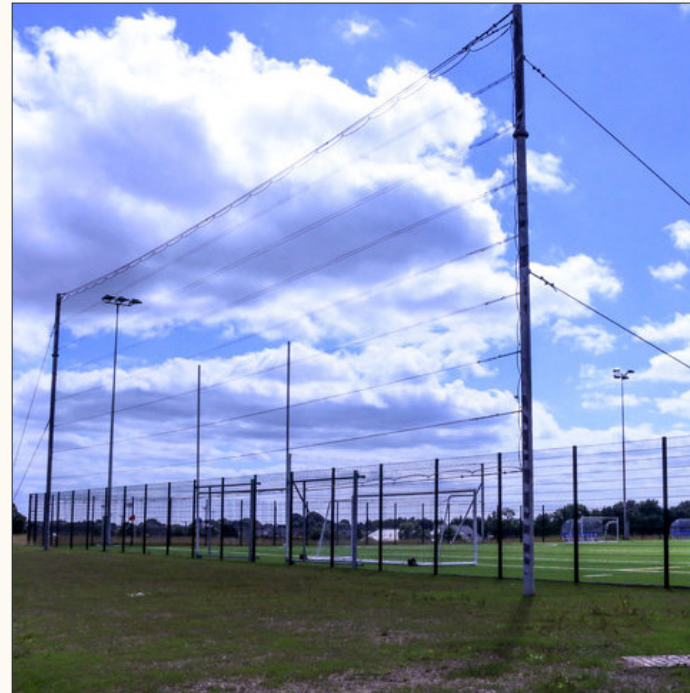
ii Typical view of ball stop nets, with 2 main stay poles and a fold up netting system.
