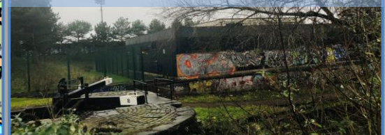
Looking across the Ashton Canal and towpath towards the site's north-eastern boundary
