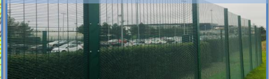
A tall, welded-wire, mesh fence secures the Campus and its North Car Park
