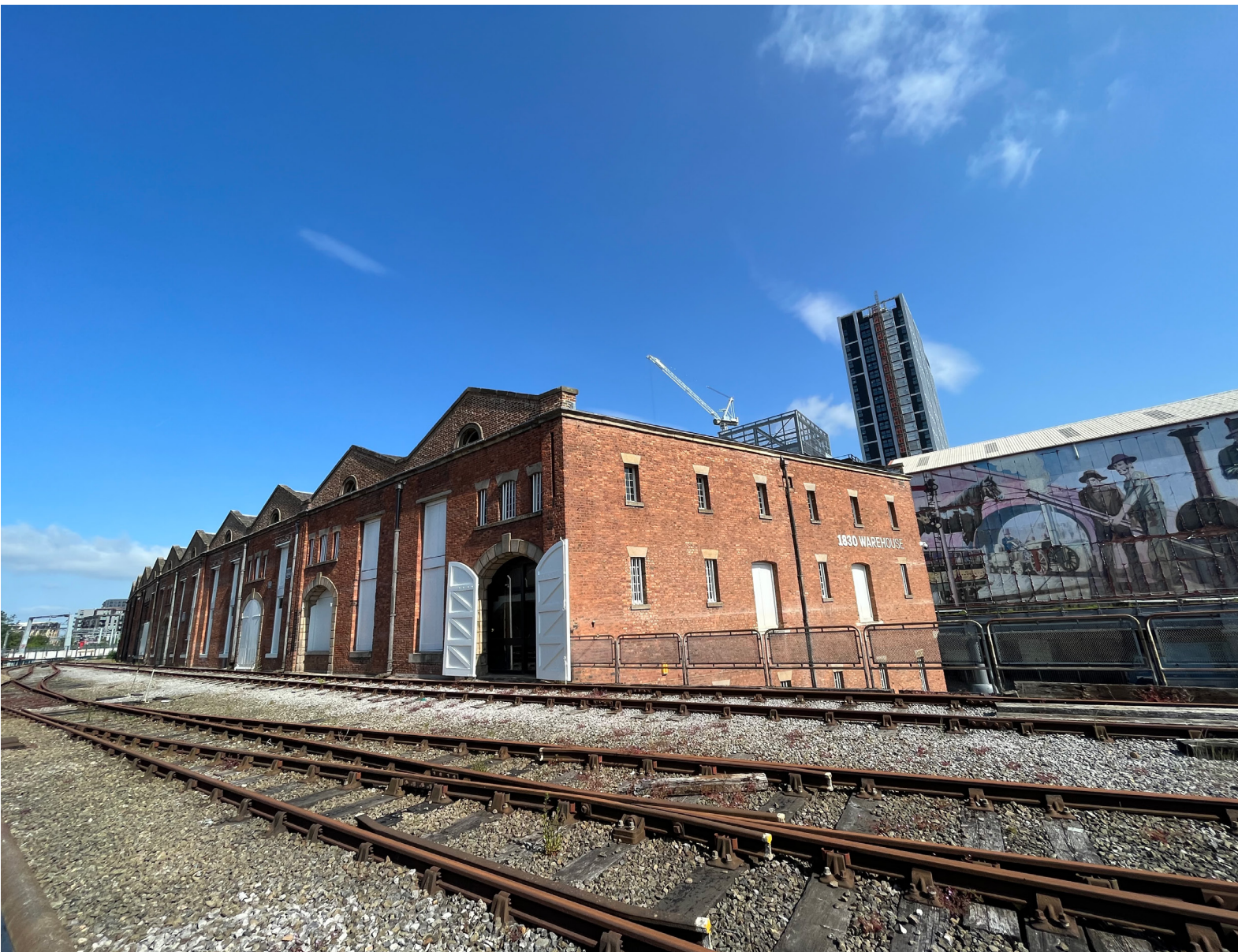
Figure 12 Southern and Eastern Elevations of the 1830 Warehouse with viaduct in the foreground
