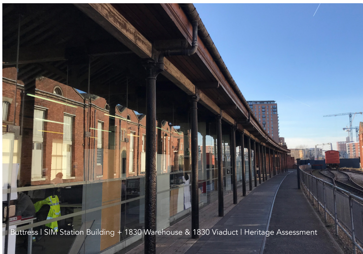
Figure 6 Top: Coach Offices to the rear of the Station Building
