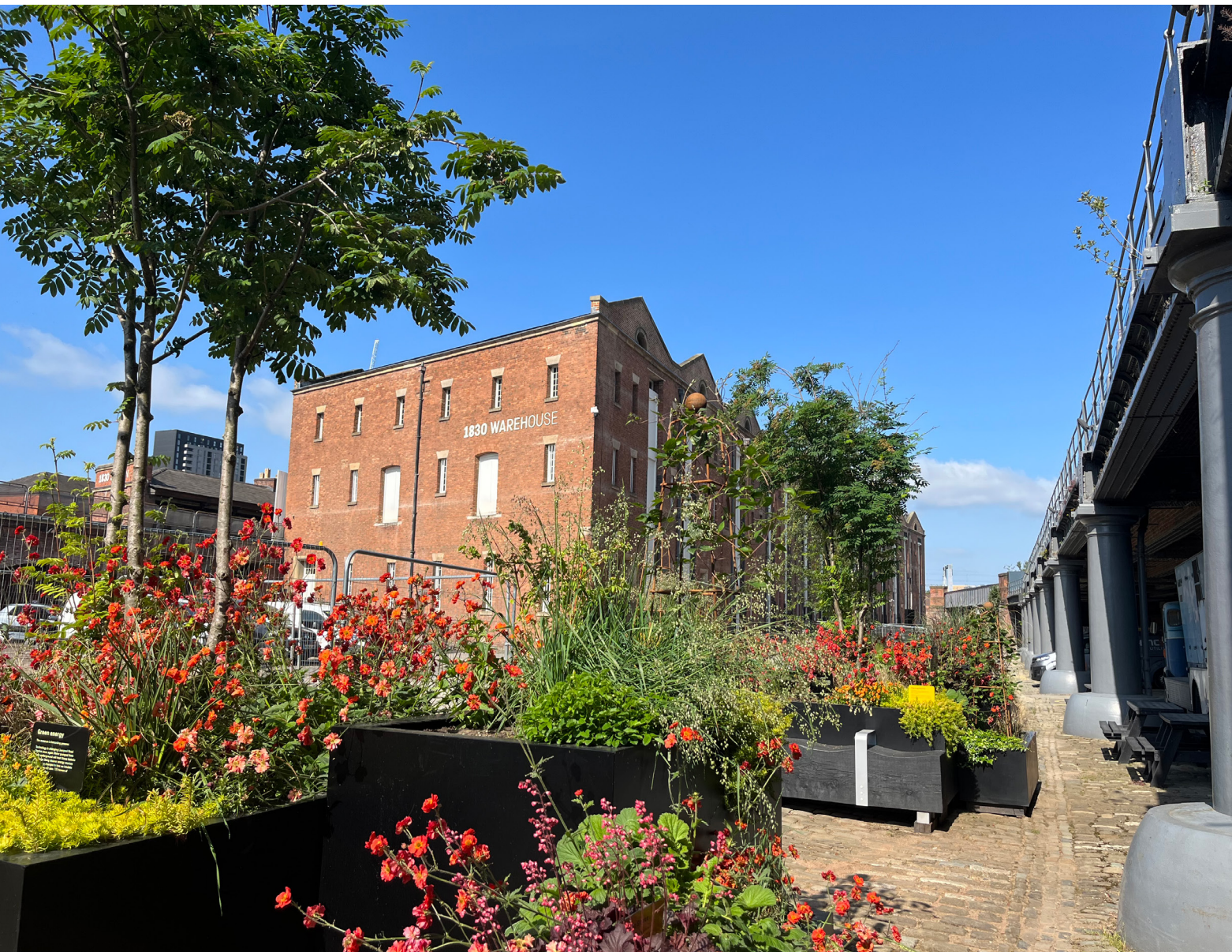
Figure 11 1830 Warehouse from lower yard
