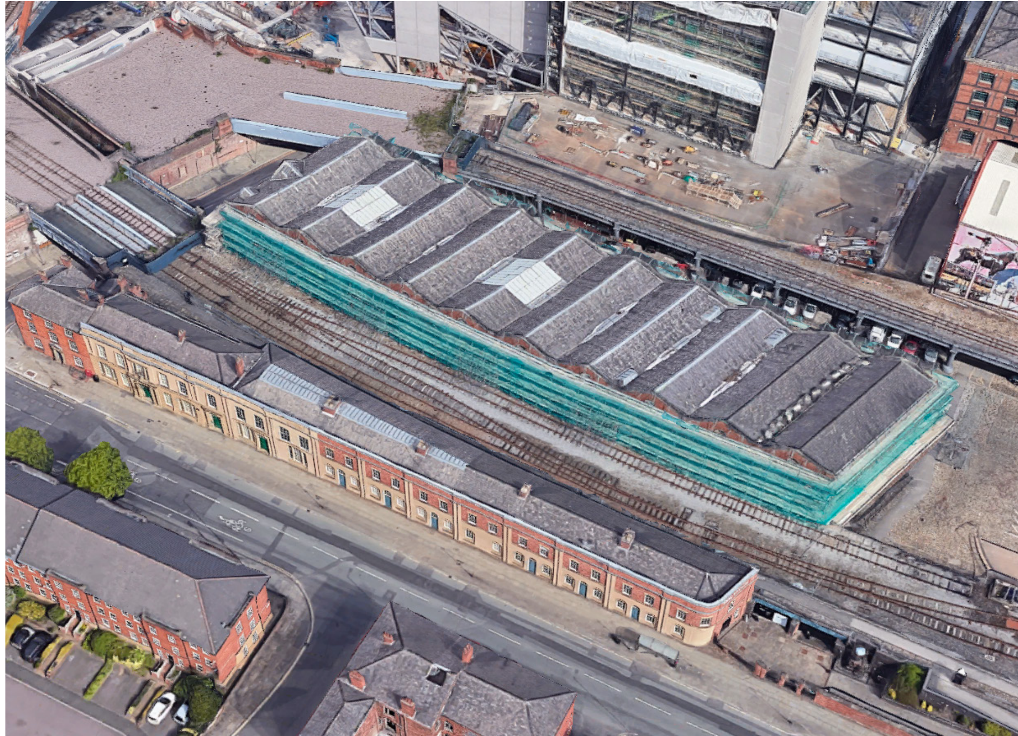
Figure 5 View of the Liverpool Road Station Complex
