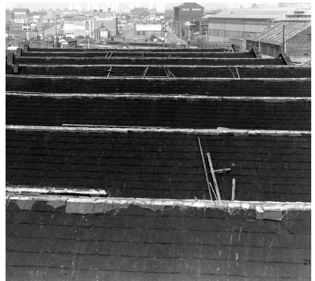
Figure 21 Top : 1830 Warehouse, 1986 © Manchester Libraries (m59048).
