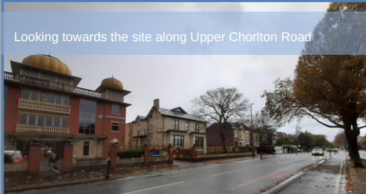
The front elevation of 63-65 Upper Chorlton Road
