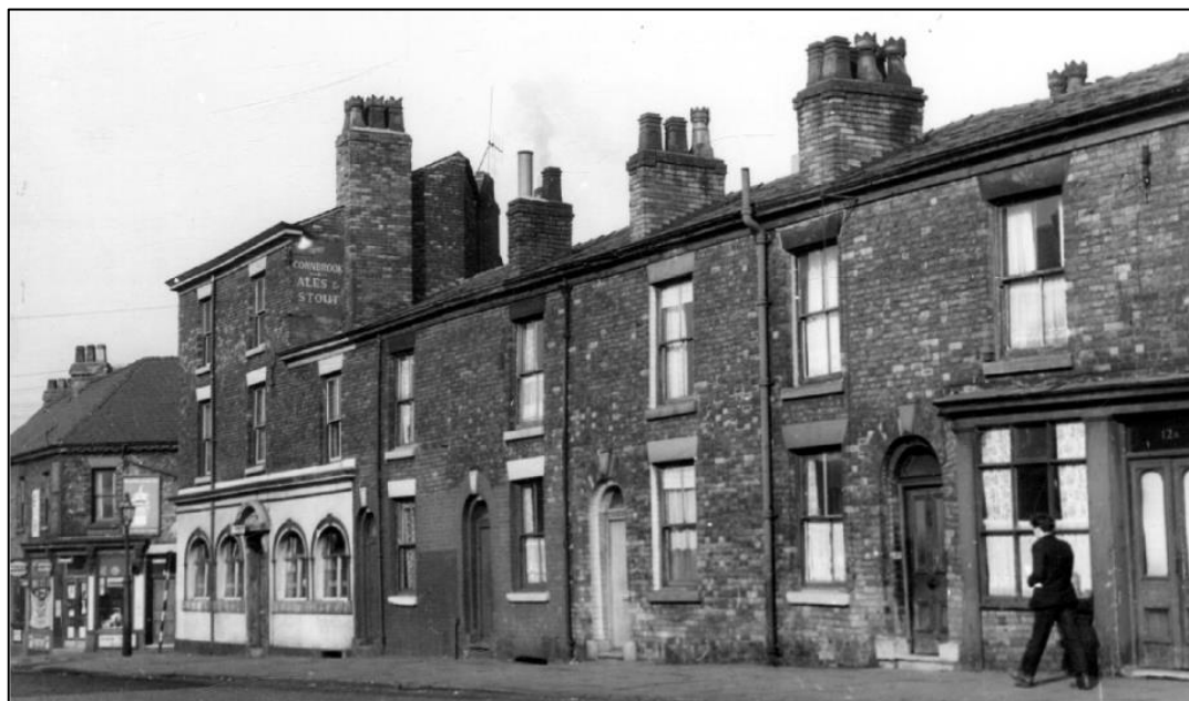
Plate 7 Houses of Cornbrook Road, 1962
