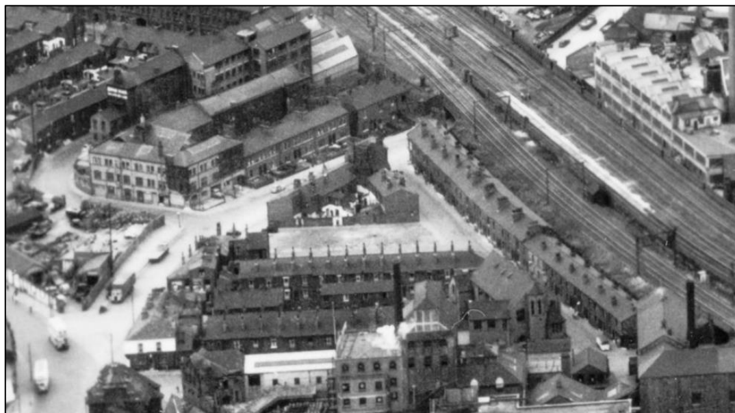
Plate 5 Area of the site looking towards Manchester Docks from the north-east, 1951
