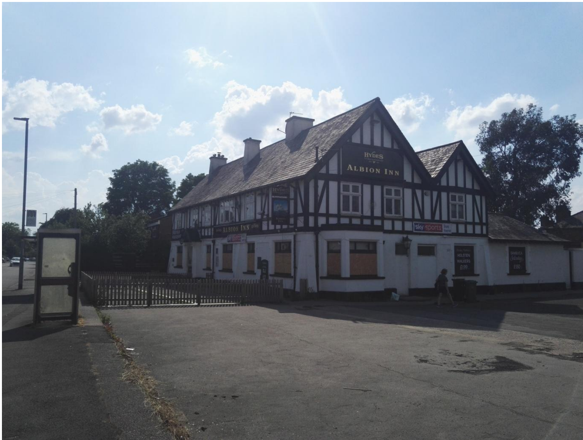
Corner Front View to Burnage Lane & Barcicroft Road
