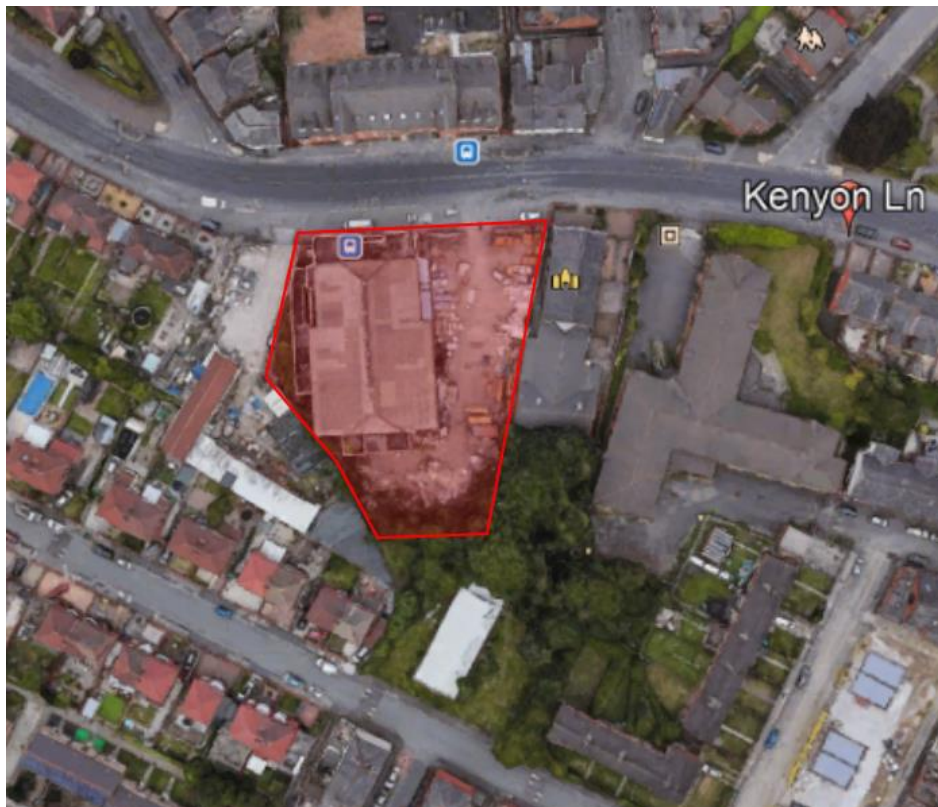
Figure 1 – Site Location (Google Maps)
